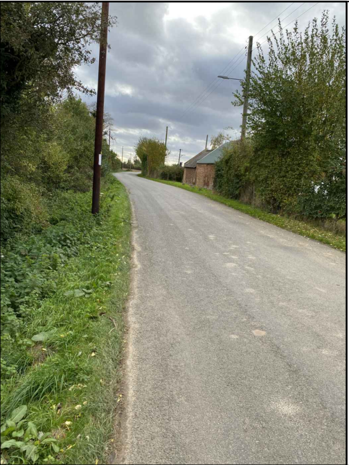
C02 Potential Asbestos
