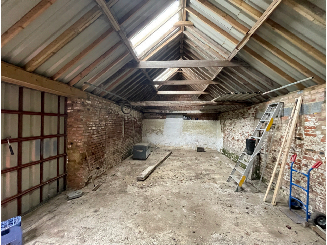
Image 4.0: View internal to newer section of Barn.
