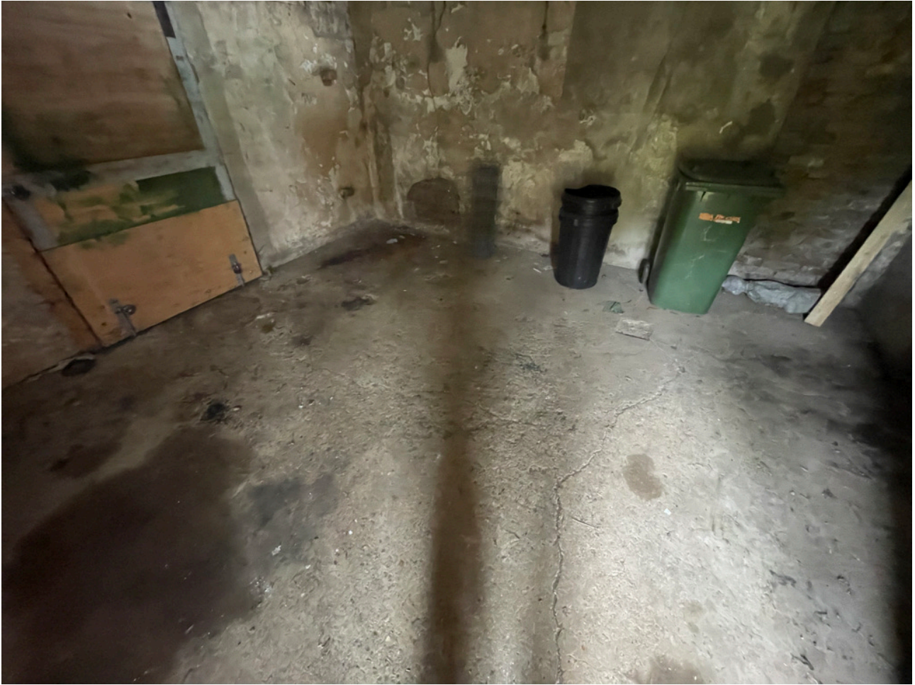
Image 20.0: Concrete slab to main barn.
