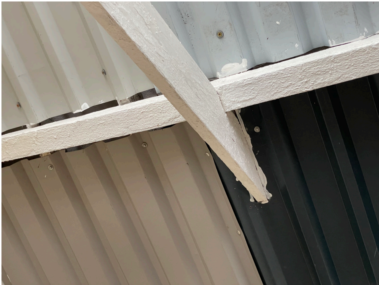
Image 6.0: Purlin, correctly restrained by ceiling binder
