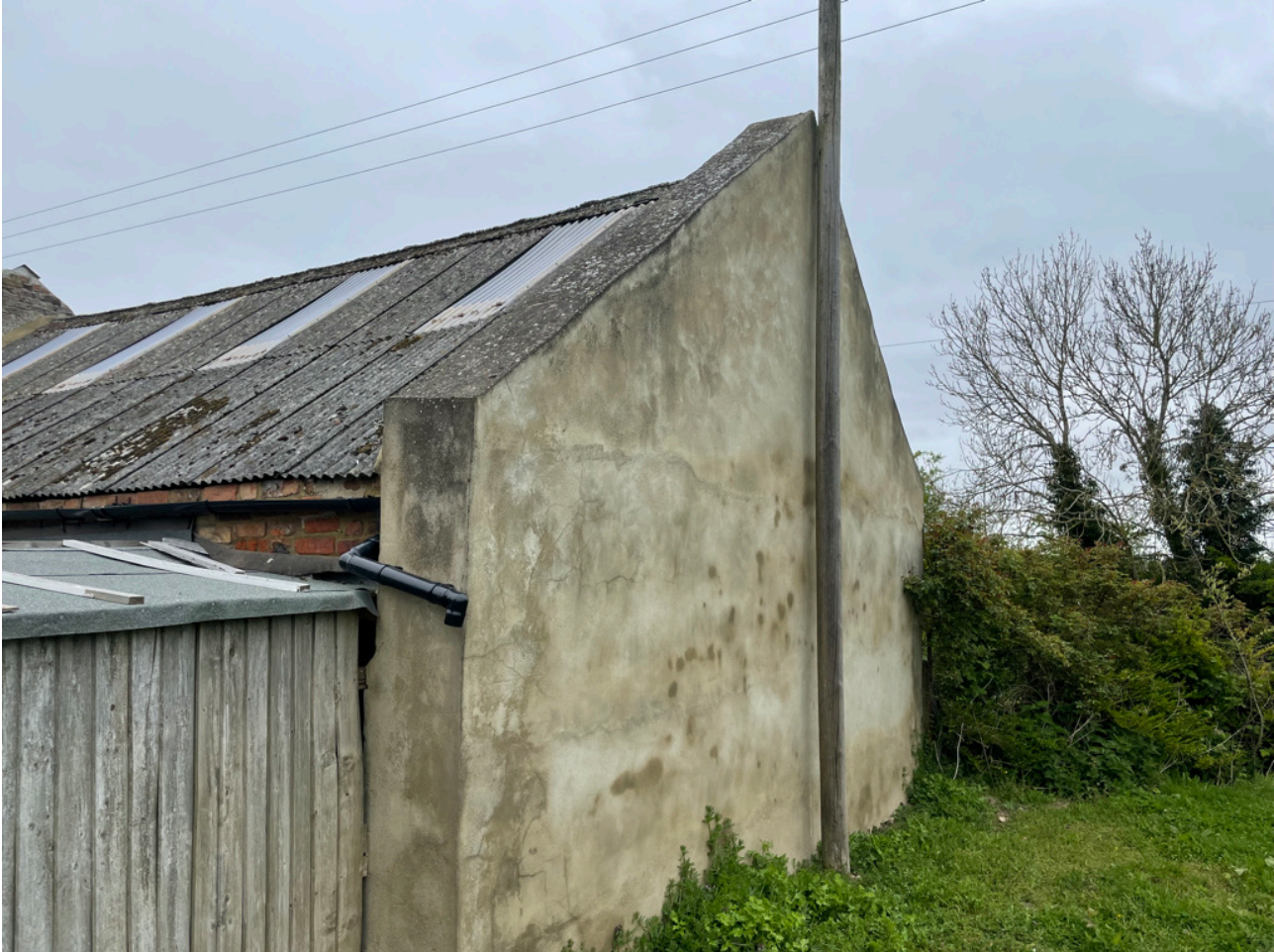
Image 10.0: External view of Gable
