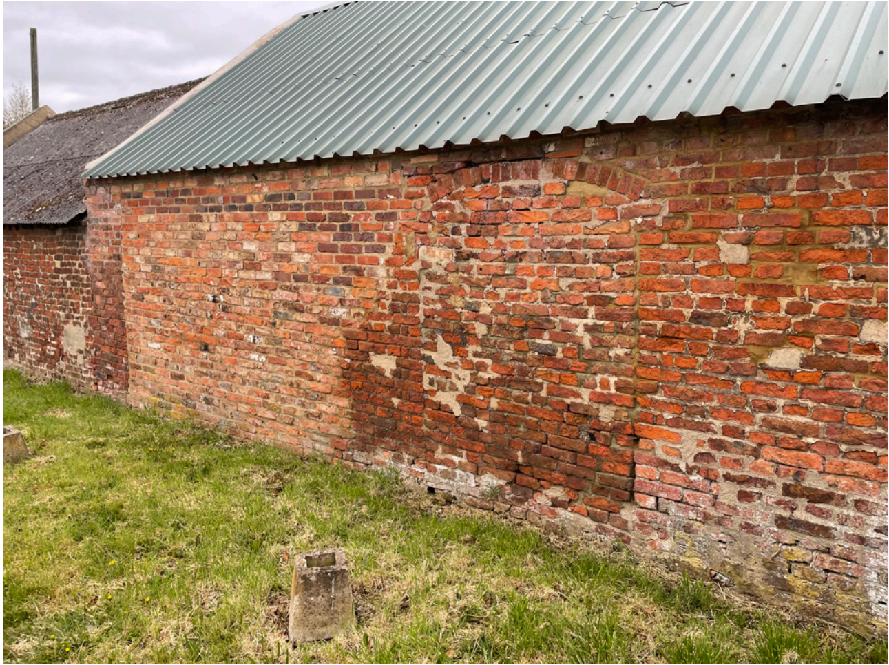
Image 2.0: Masonry arch to head of former opening, now infilled.
