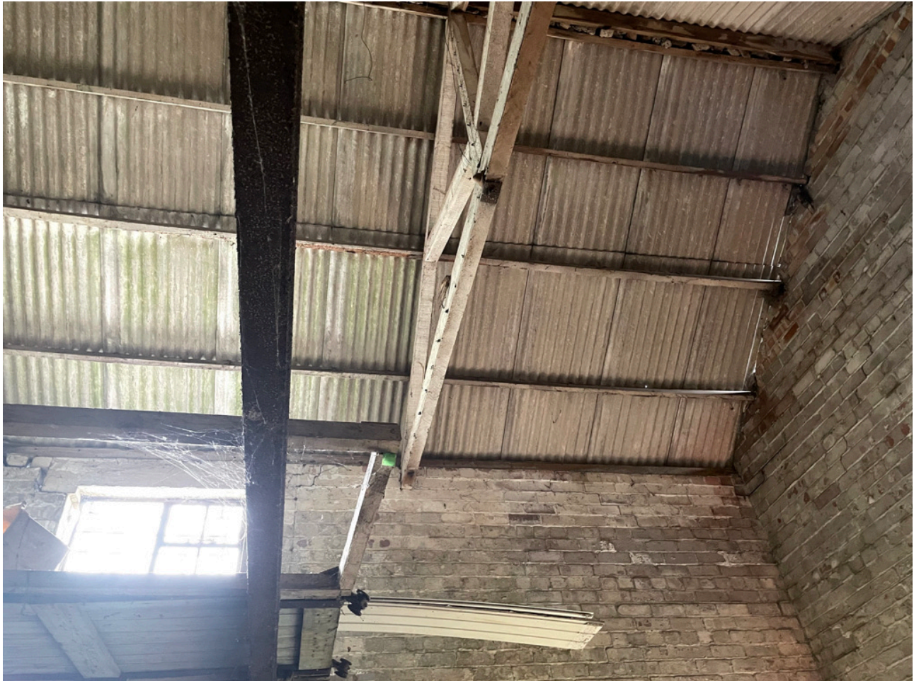
Image 13.0: Purlins to underside of corrugated cement roofing sheets
