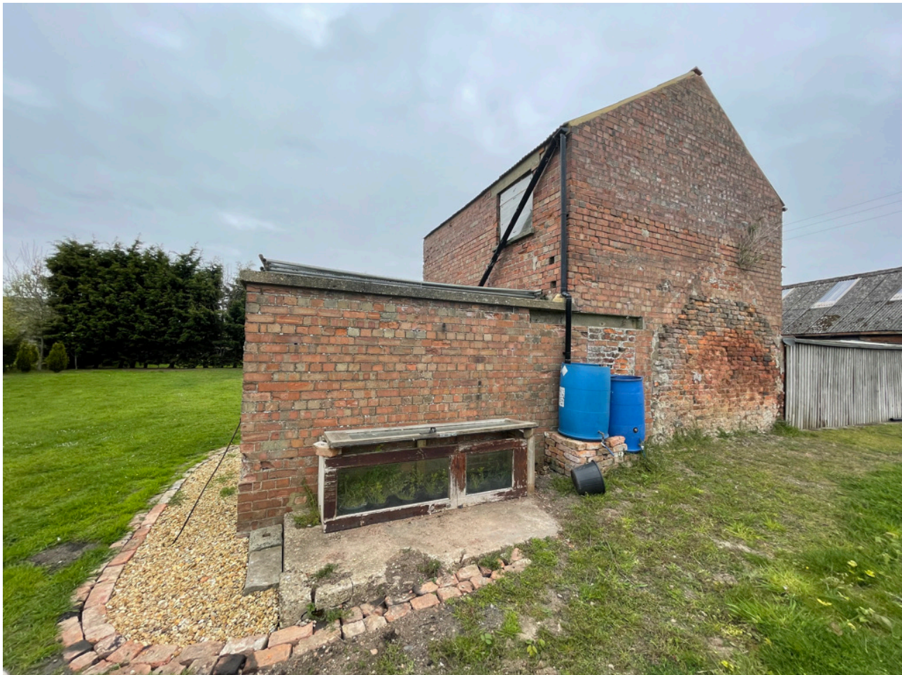
Image 12.0: Two storey structure with single storey extension.
