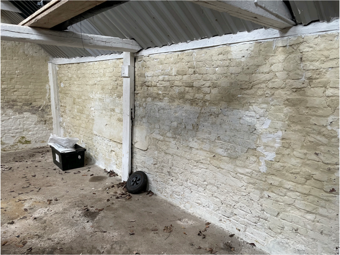
Image 7.0: View of side wall and finished floor
