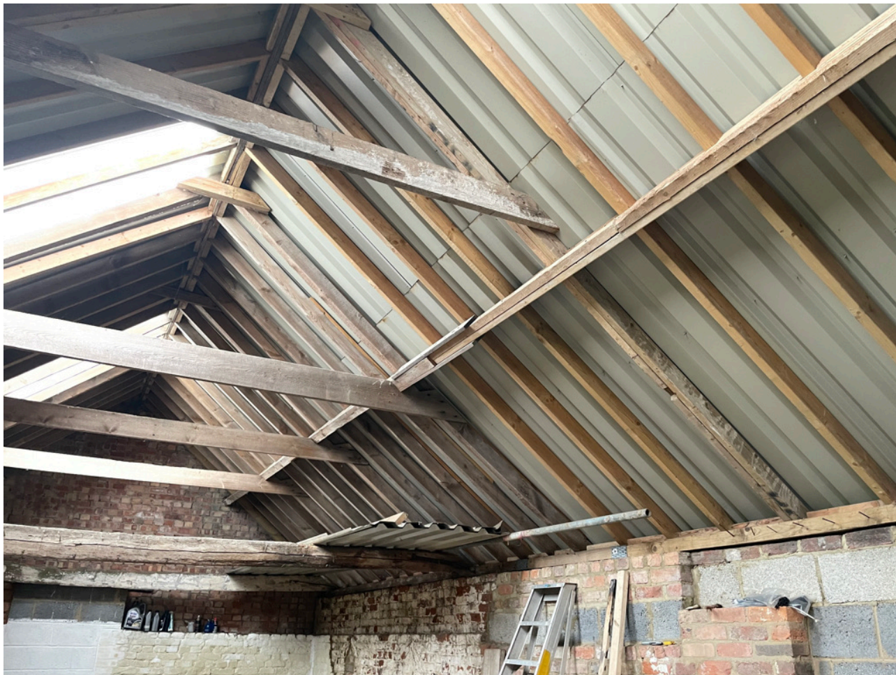
Image 3.0: Roof structure to newer section of barn with corrugated steel sheeting
