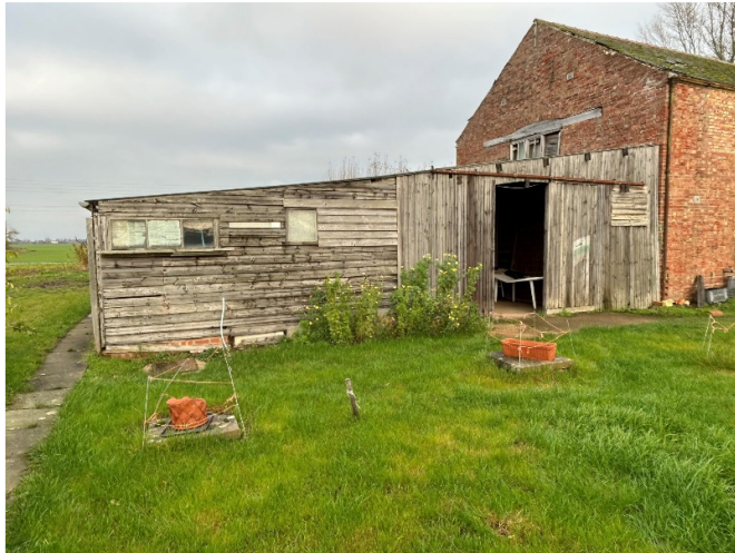
Pic 8 - South-east facing elevation of attached timber storage area
