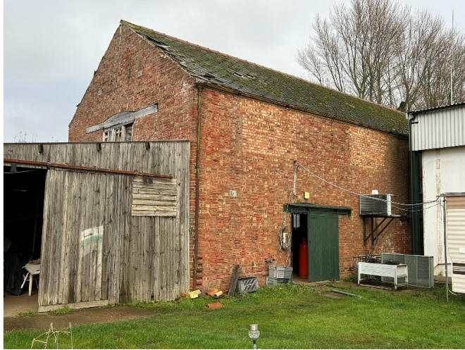
Pic 5 - South-east facing wall (side) Elevation
