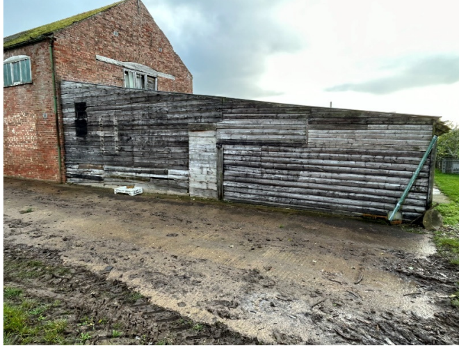
Pic 7 – North-west facing elevation of attached timber storage area
