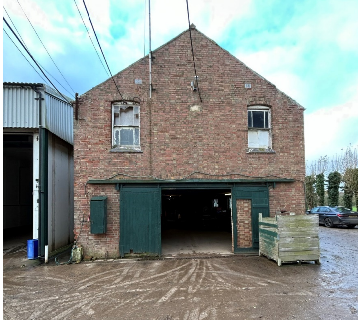
Pic 4 - North-east facing wall (gable) Elevation
