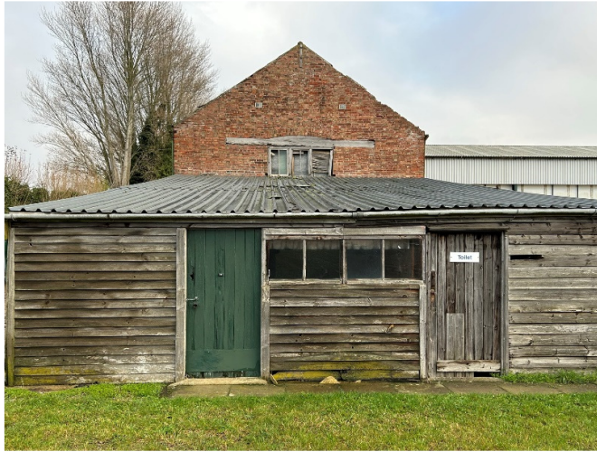
Pic 6 - South-west facing wall (gable) Elevation
