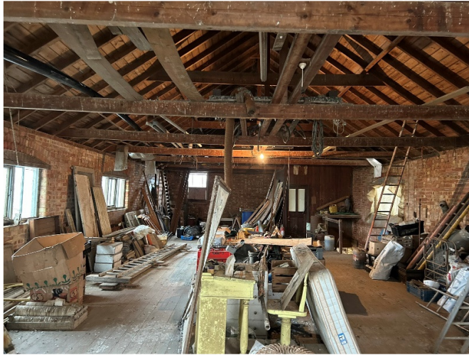
Pic 10 – Roof structure – General view
