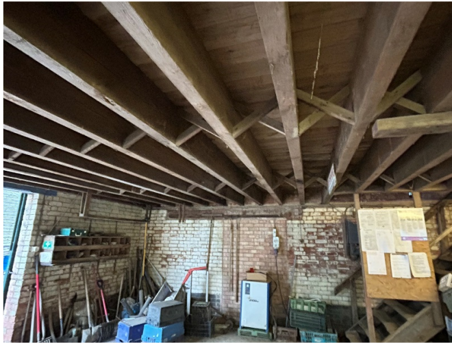
Pic 9 – Underside of first floor (showing herring bone strutting)
