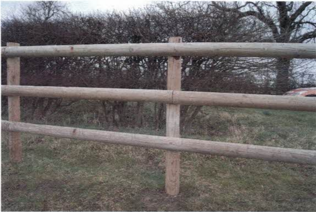
Photo 3 – Post and Rail Fencing 1.2m high (approx.)
