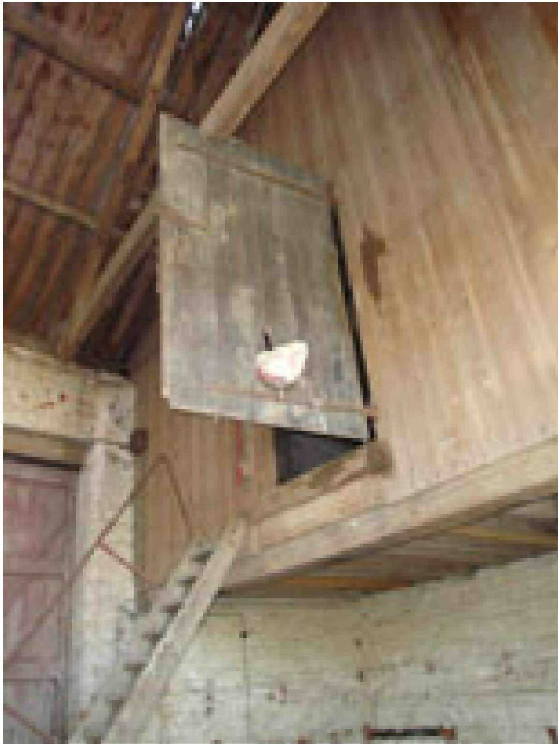
Hay Loft Mezzanine - Photo B
