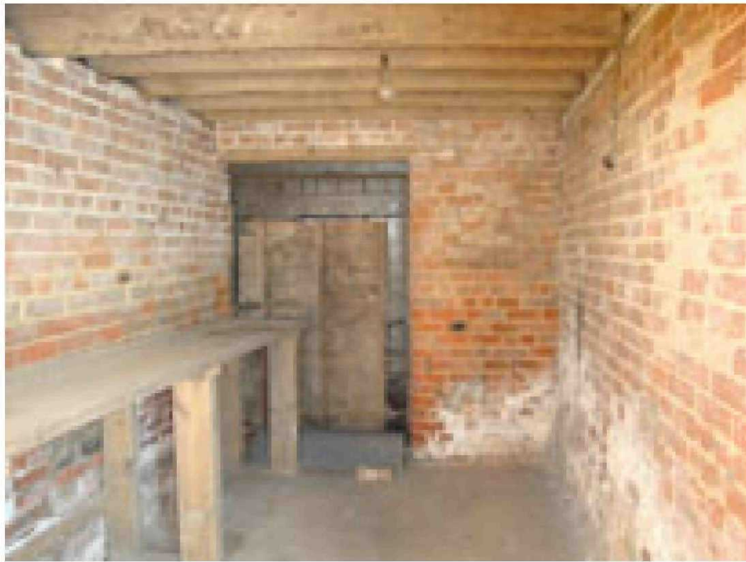
Ceiling Timbers over Store - Photo A
