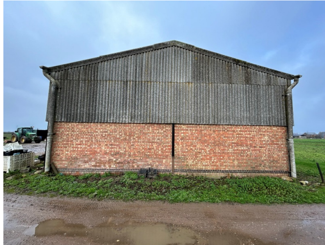
Pic 4 - South-east facing wall (gable) Elevation
