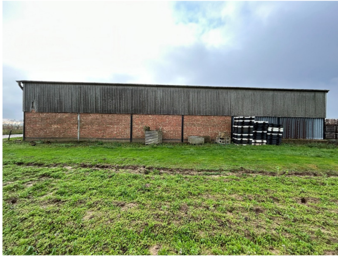
Pic 5 - North-east facing wall (side) Elevation
