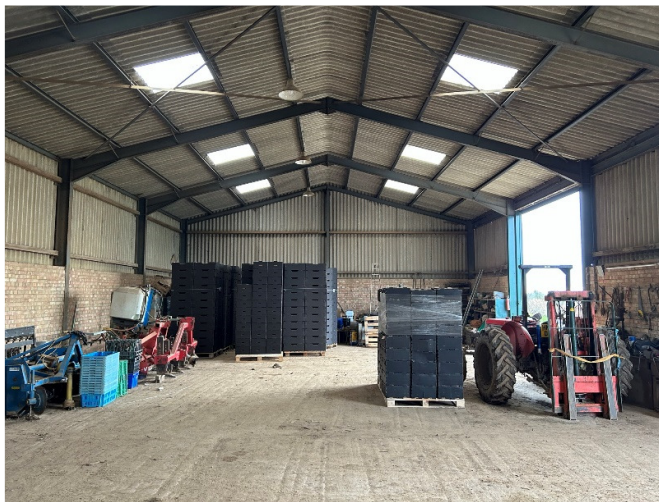
Pic 7 – General internal view of Steel Framed Barn
