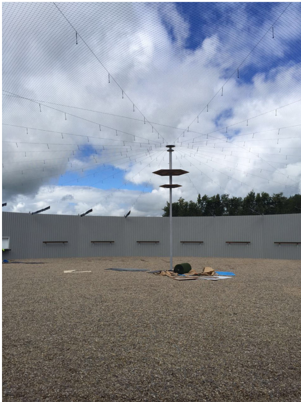
View showing gravel ground, corrugated metal walls, central pole and netting above
