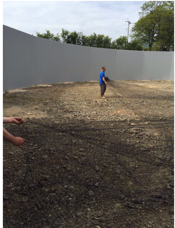
View of netting being spread out for installation
