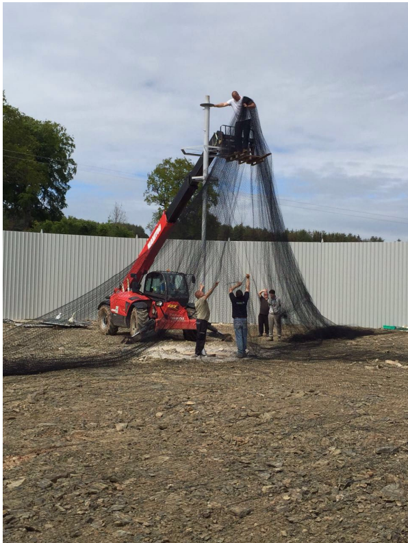
View of central pole with netting being installed
