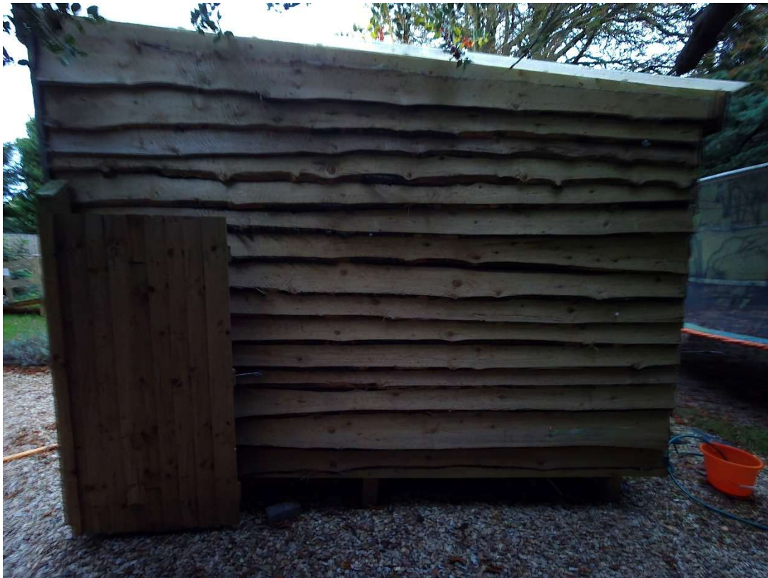
Timber Structure – Side Elevation (West)
