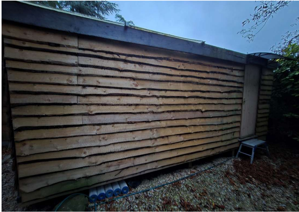
Timber Structure – Rear Elevation (South)
