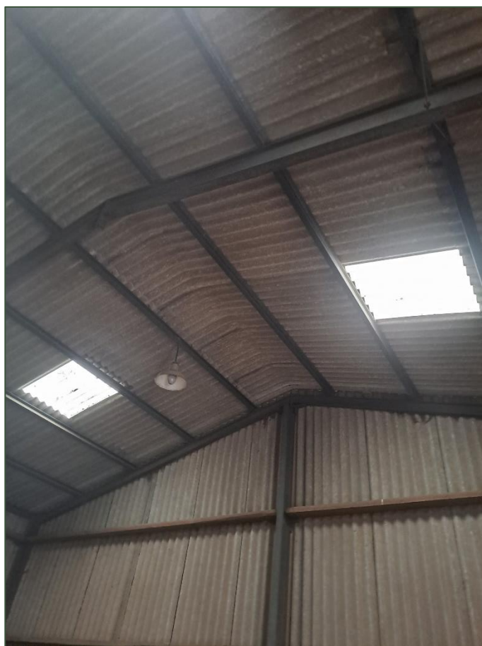
Plate 7 – View of the barn interior.
