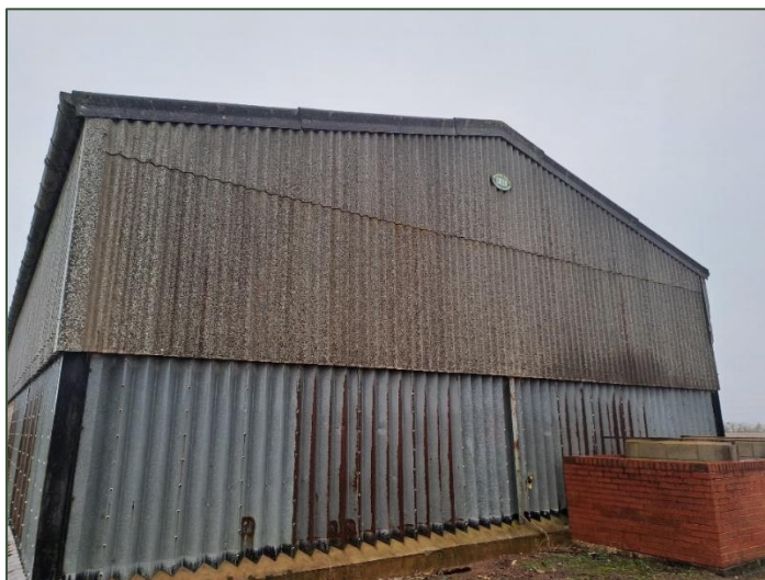
Plate 6 – View of the barn exterior.
