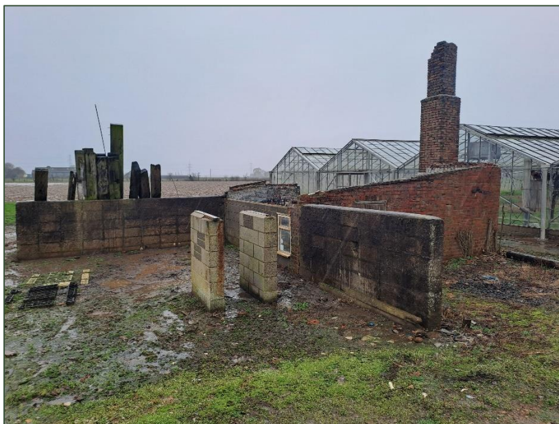
Plate 5 – View of the ruined boiler-house.
