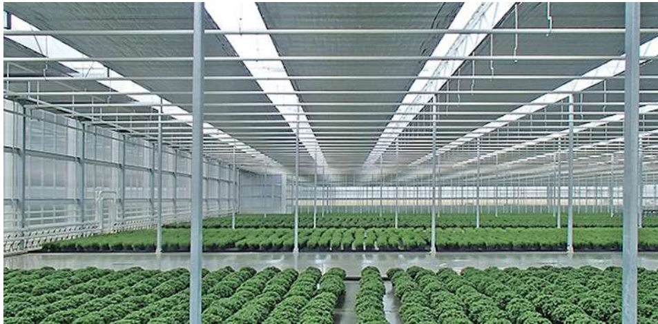
Figure 10 Typical Glasshouse Blackout Blind System
