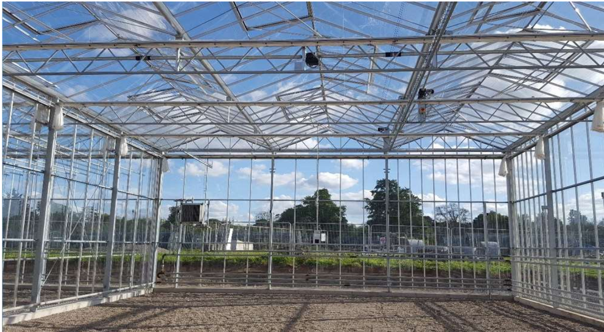
Figure 8 Typical Glasshouse Structure
