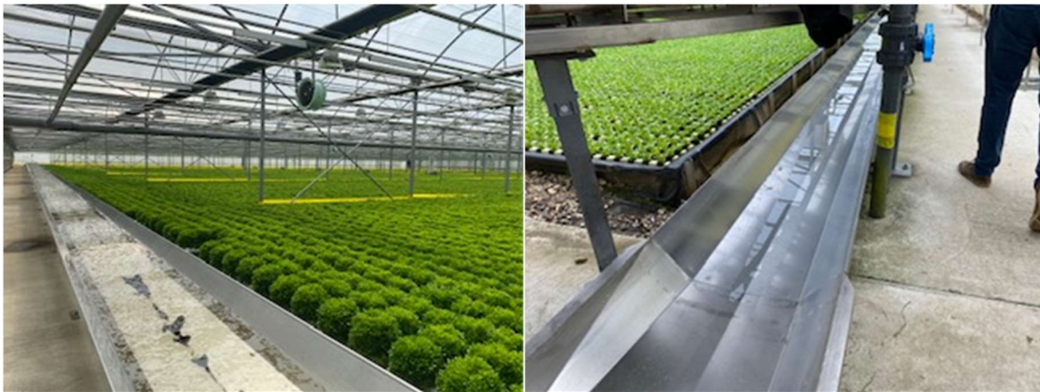
Figure 9 Typical Glasshouse Structure
