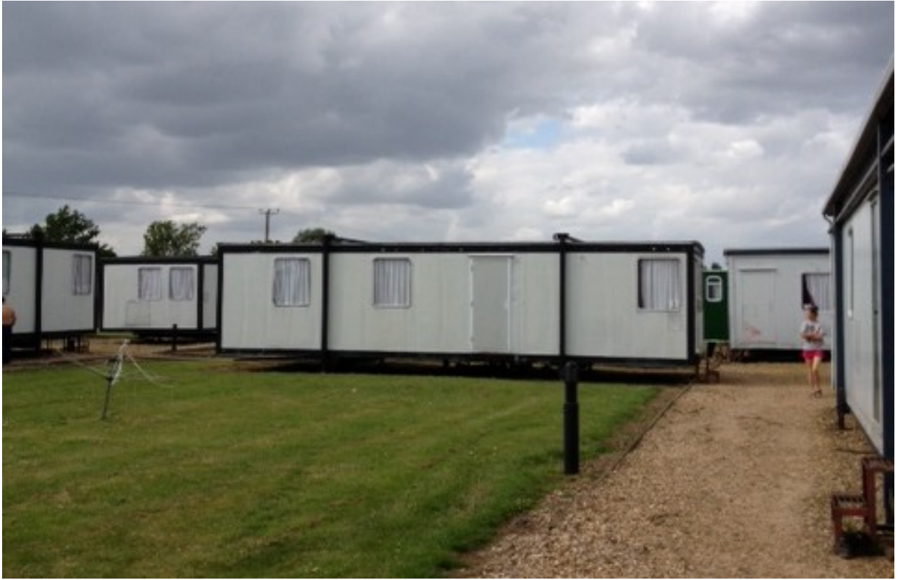
Portcabins at Onslow Camp
