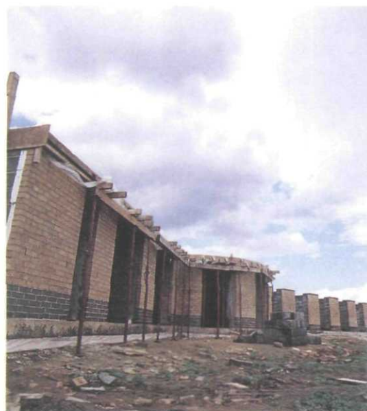
LEFT AND ABOVE: Work on the house continues. The doorway above is designed to aid air flow through the house from the warm south-facing side to the cooler north side. Passive ventilation is the main form of cooling for the building.
