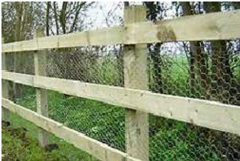
Post & 3 rail (wire stockproof) fence
