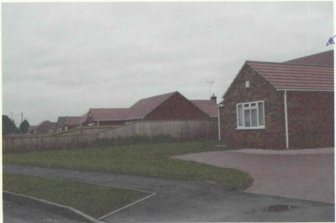
view north from road with site off picture to right
