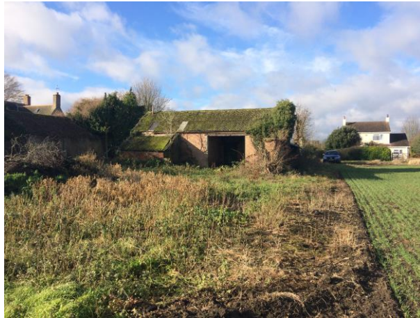
Existing Barn 1 Rear
