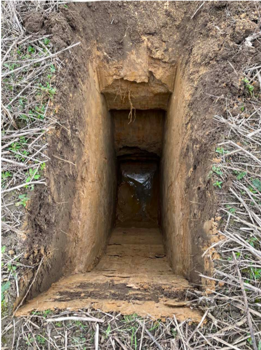
Image 6.0: View toward base of trial pit 3, with liquefaction of base due to ground water infiltration.
