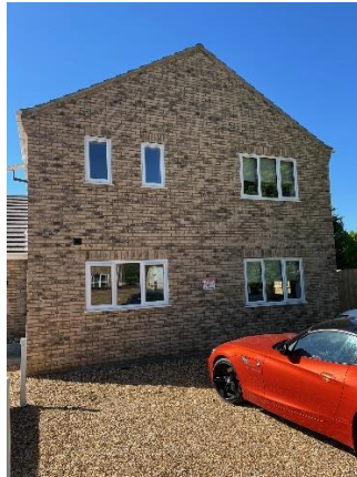
Existing Two Storey Element of Clubhouse to be converted
