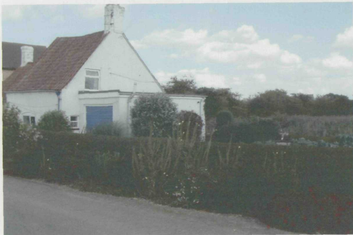
looking across road north onto no 25
