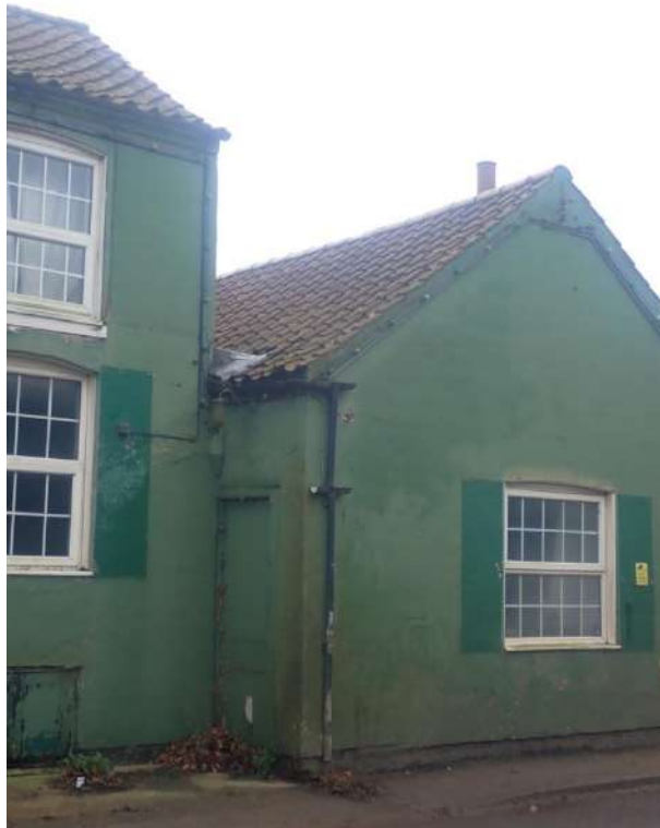
Plate 282: View of Building 3, from the north-east
