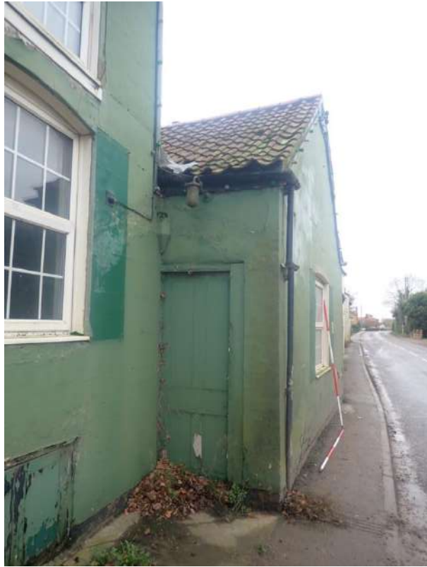
Plate 283: View of Building 3, from the north-east
