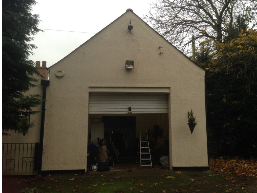
Front of Threshing Barn
