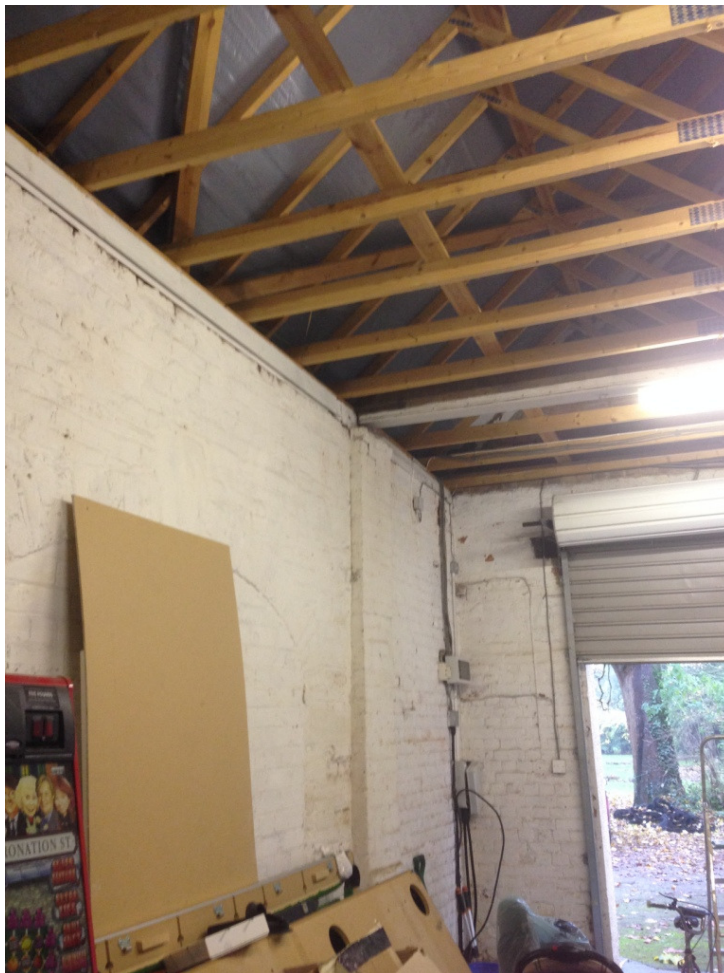
Brick arch visible inside the barn
