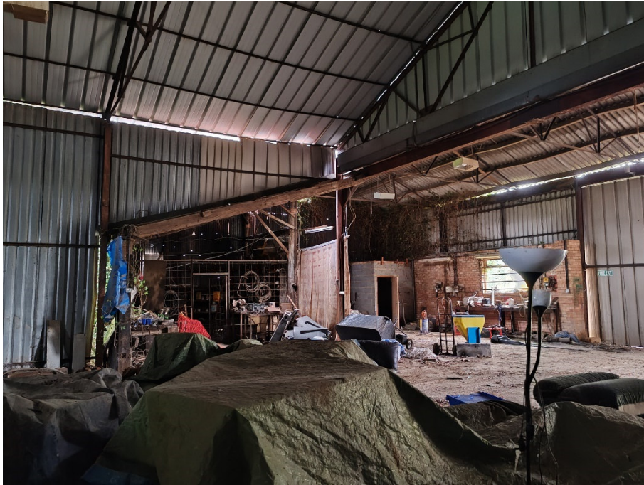
Site walkover photo: 8 Date: 05 Aug 2024 Photo direction: West Description: View inside of barn and stored wares including furniture and carpentry tools
