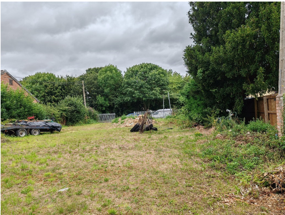
Site works photo: 1 Date: 05 Aug 2024 Photo direction: North Description: View of existing grassed yard, scrub vegetation and stockpiles
