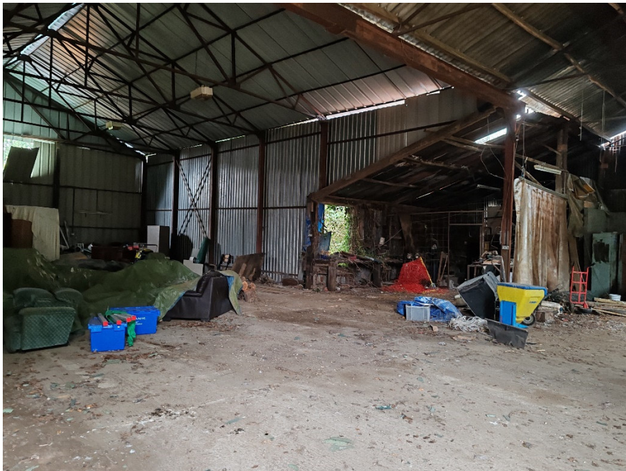
Site walkover photo: 5 Date: 05 Aug 2024 Photo direction: Southwest Description: View inside of barn with miscellaneous items such as sofas and bins
