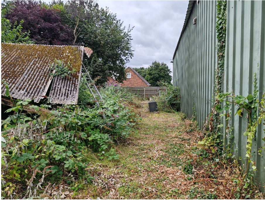
Site walkover photo: 4 Date: 05 Aug 2024 Photo direction: South Description: View of side of barn, disused cattle shelter and surrounding overgrown vegetation
