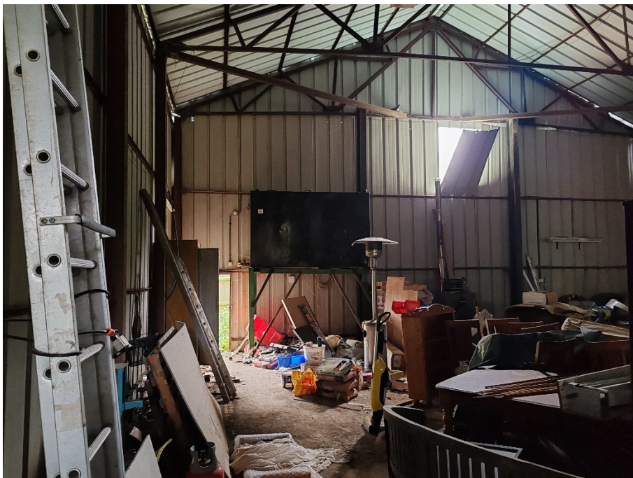
Site walkover photo: 9 Date: 05 Aug 2024 Photo direction: South Description: View of inside of barn with assorted wares, red diesel tank and possible asbestos roof
