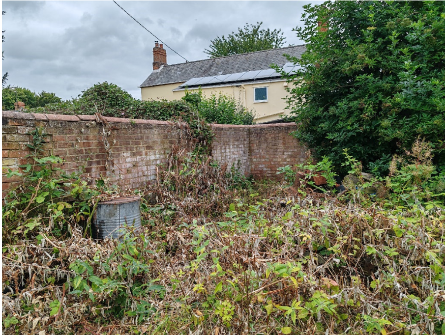
Site walkover photo: 12 Date: 05 Aug 2024 Photo direction: Southeast Description: View of overgrown garden area behind barn
