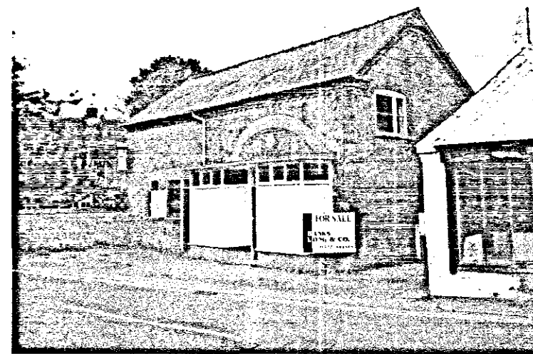
Ph 02 - General exterior view
