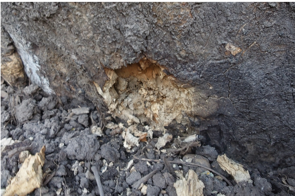
Decay in exposed heartwood
