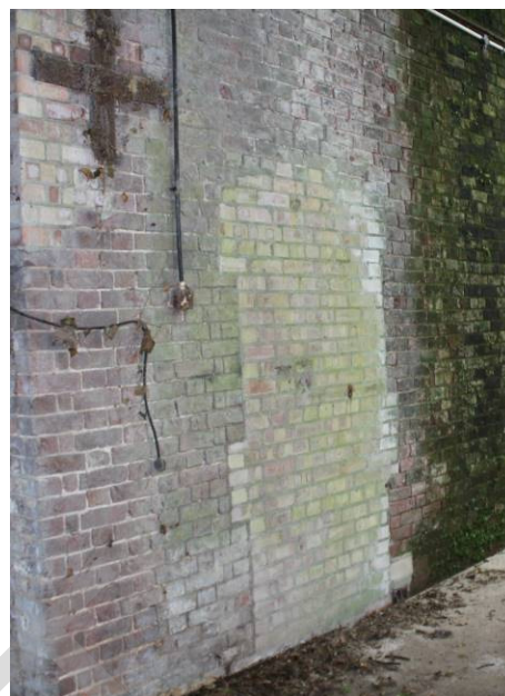
Plate 9 (above). Blocked door, northeast end of the southwest elevation of the threshing barn
