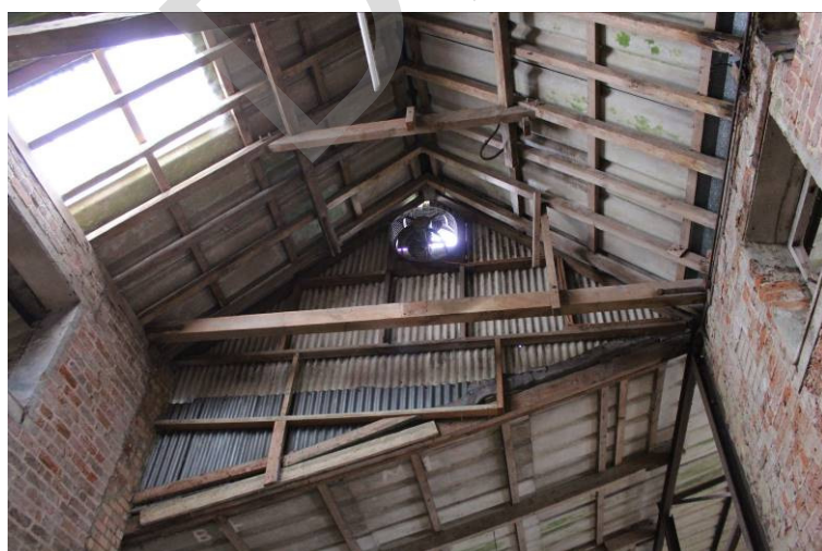
Plate 17. Detail of the roof timbers over the removed southeast gable end of the threshing barn
