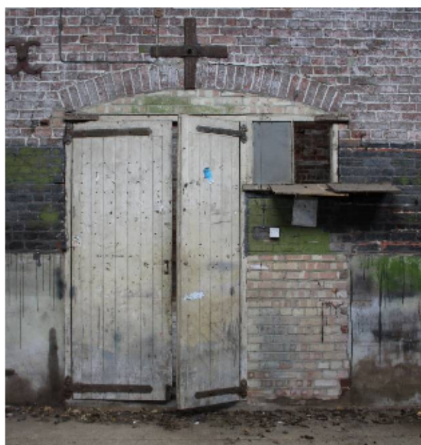
Plate 7. The wide door to the northeast elevation of the threshing barn, infilled in the 20 th century
