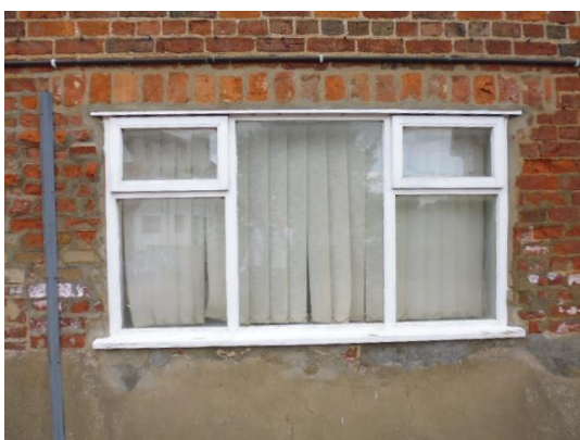
Fig. 07 – Landscape window on the east elevation
