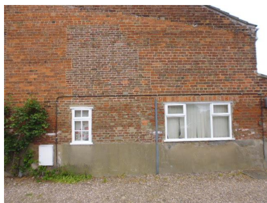
Fig. 08 – Wider view of windows on the east elevation.
