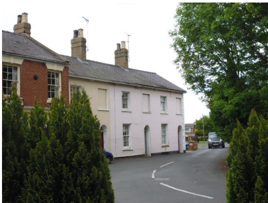
Fig. 01 – Terraced block from south (14 on right).
