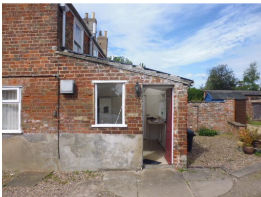
Fig. 09 – North lean-to from the east.
