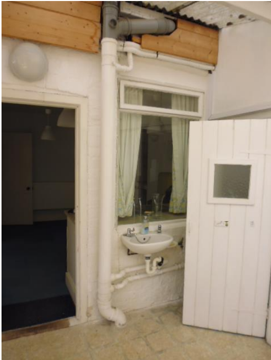
Fig. 13 – North wall at ground floor level.
