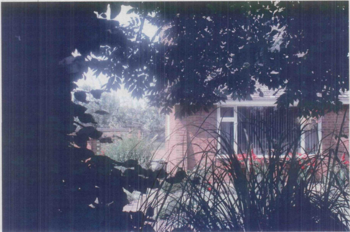
Elevation of no 59 facing no 61
