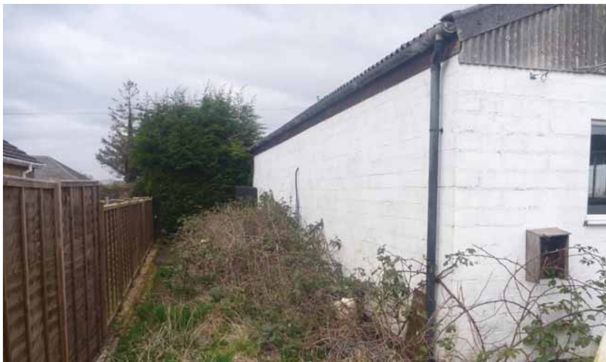
Figure 3: View west showing the retained Substation building
