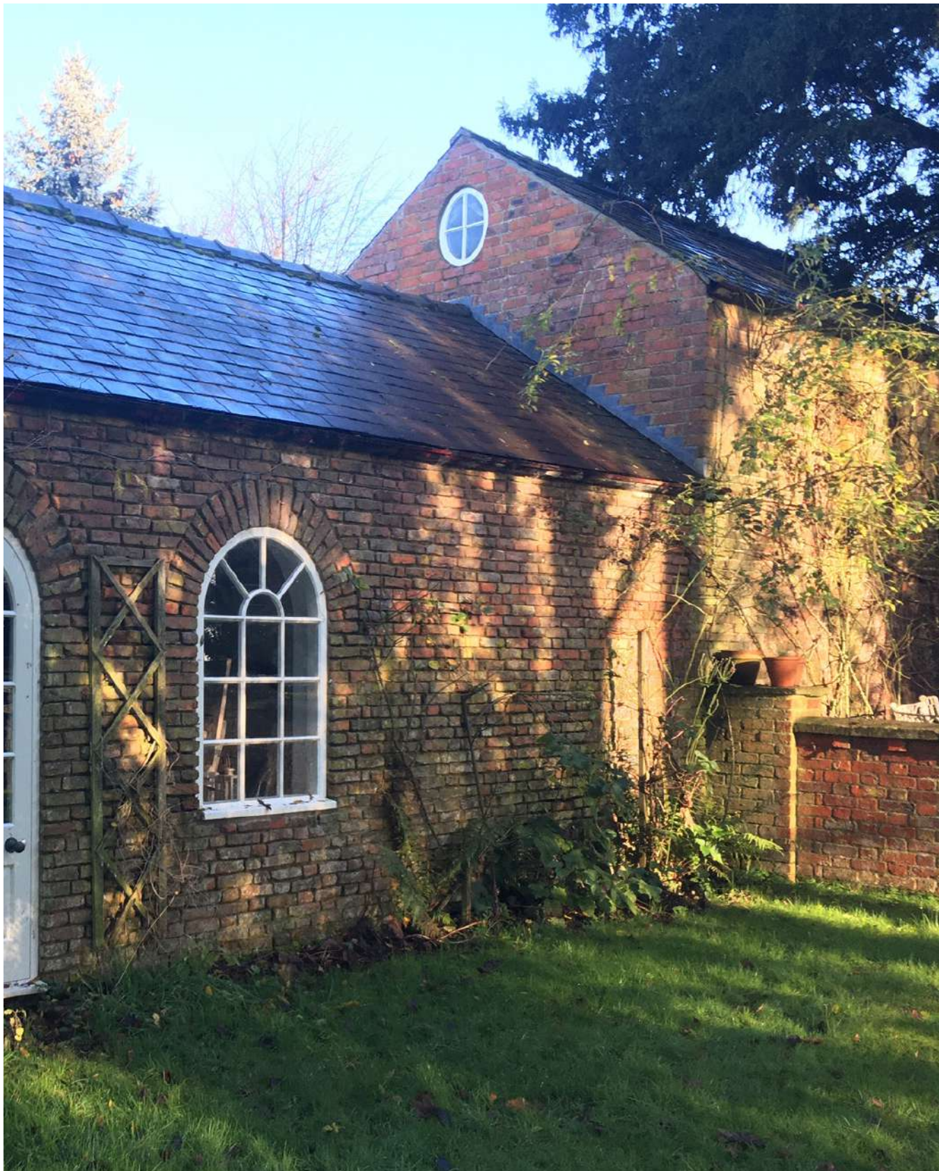
SOUTH ELEVATION EXISTING PHOTOS
