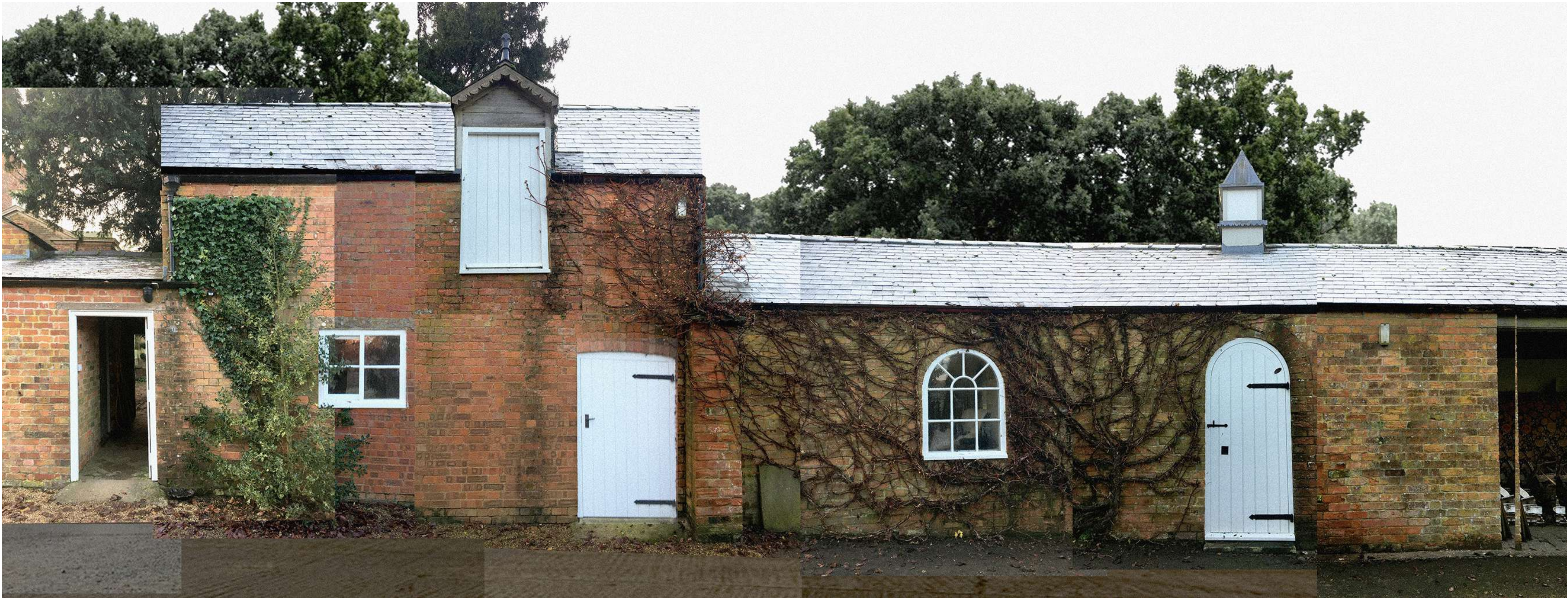
NORTH ELEVATION EXISTING PHOTO MONTAGE
