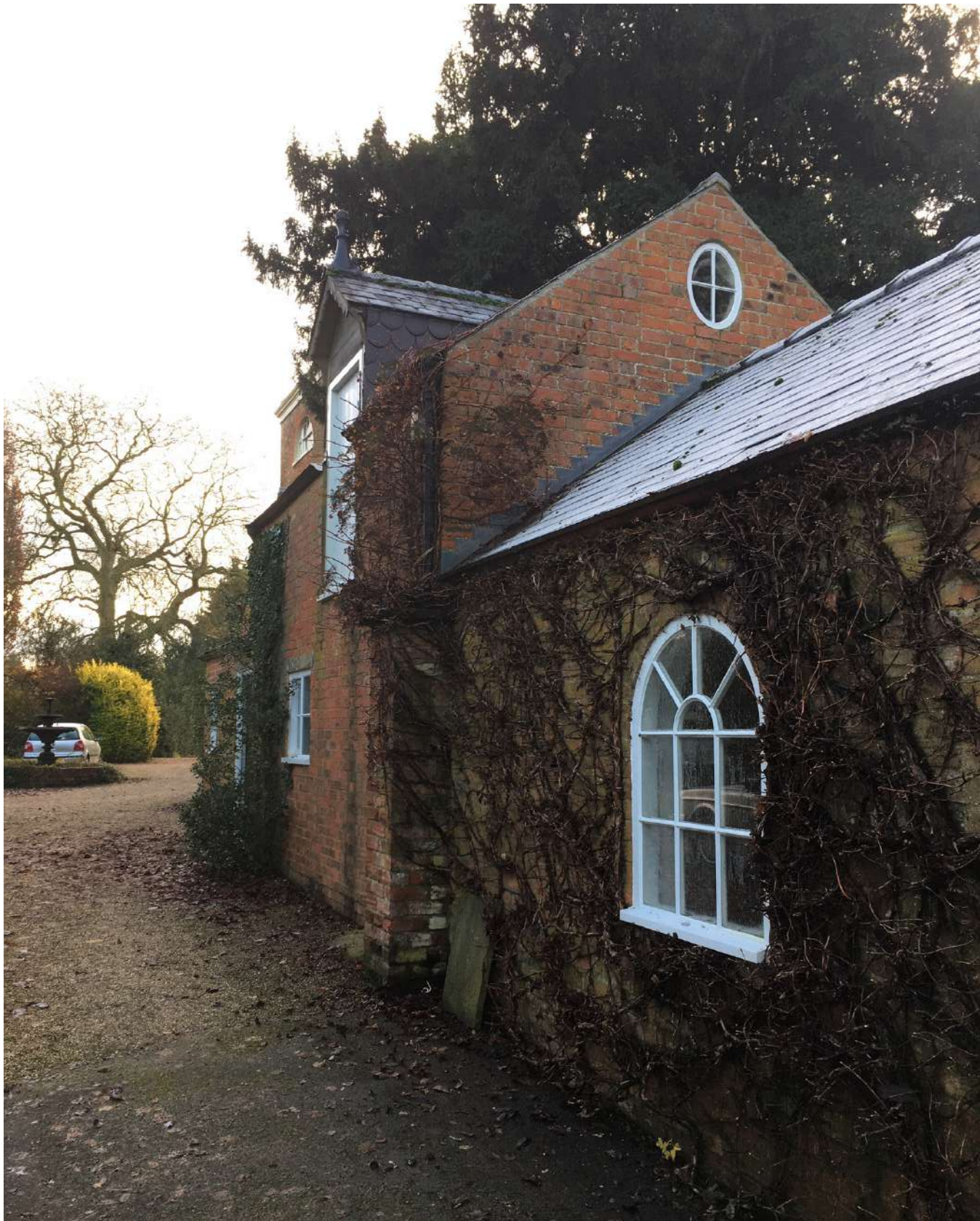
NORTH ELEVATION EXISTING PHOTOS
