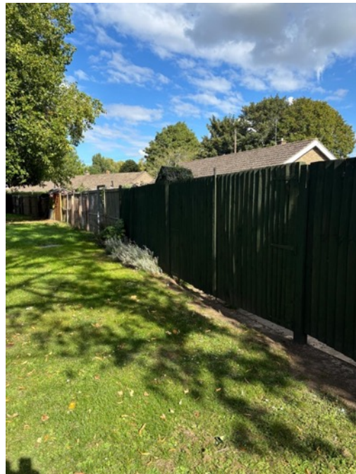
View along the east boundary
