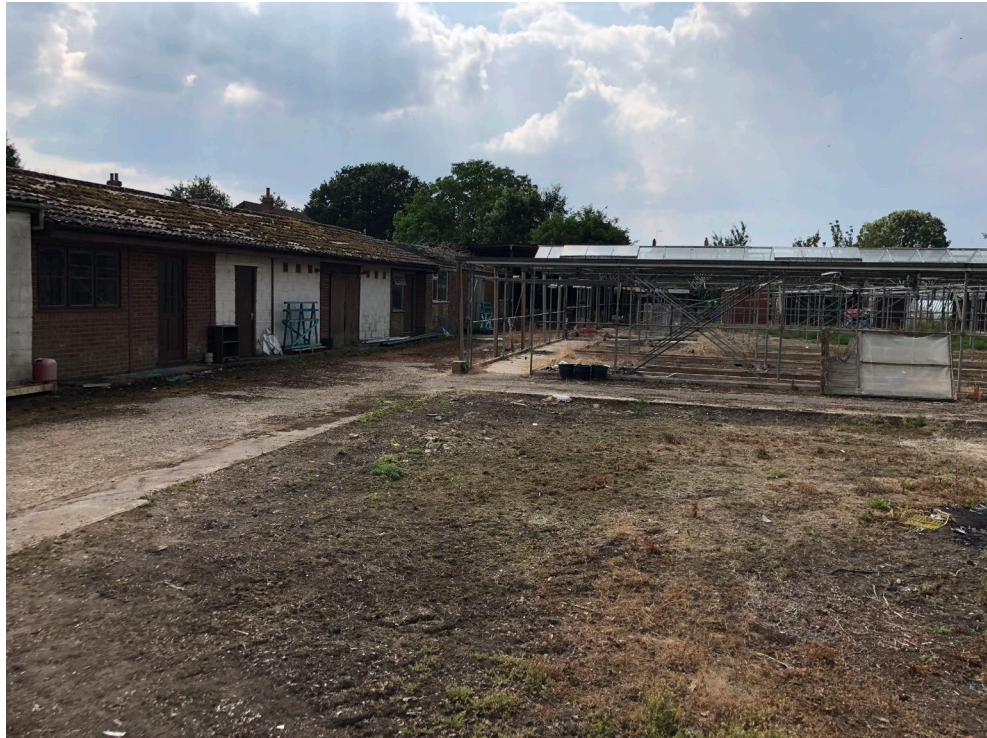
Former horticultural building with implemented planning permission to be used as a 4 bed dwelling with old glasshouses to the north
