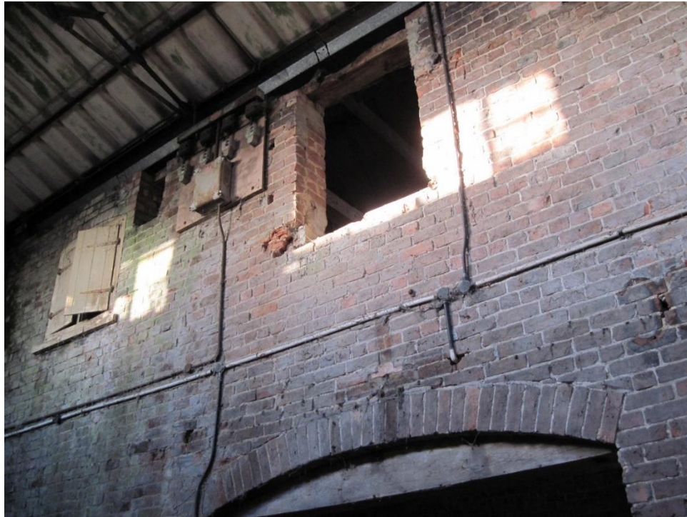
Brick arch and original architectural features
