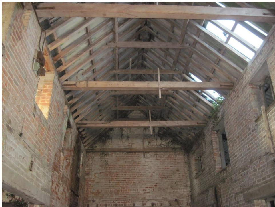
Looking at the 'barn within a barn'.
