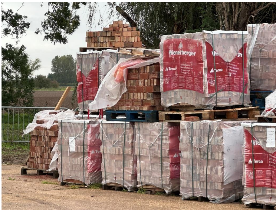
Figure 1 - Wienerberger red multi brick stock to be used to be used to construct house.
