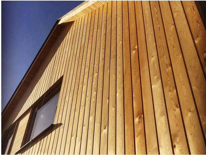
Figure 2- vertical timber cladding example
