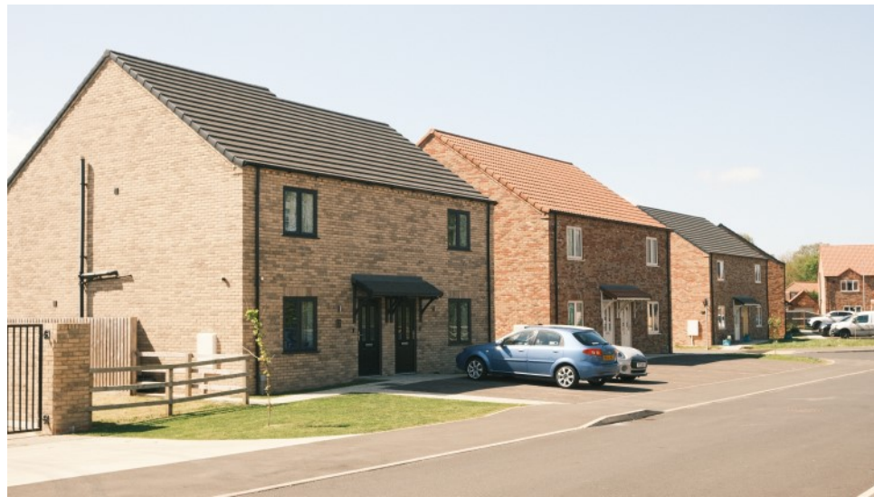
New residential development to the south of the site. The primary facing material a mix of buff and red facing brick with slate and terracotta roof tiles.
