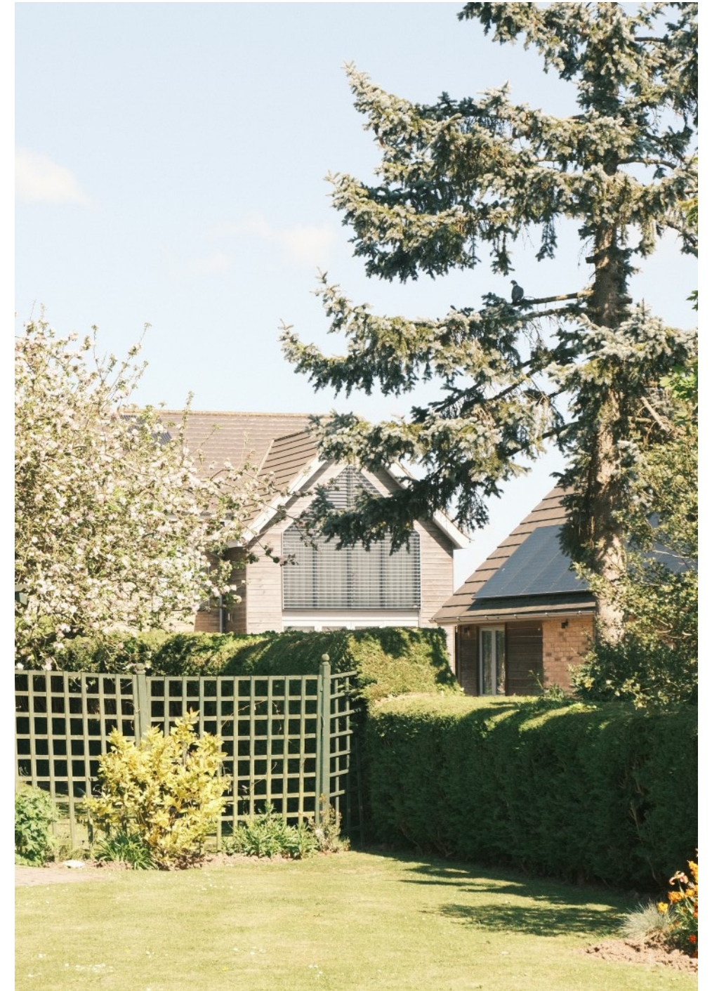
Timber Clad Gable on property adjacent to no. 43 Mill Lane
