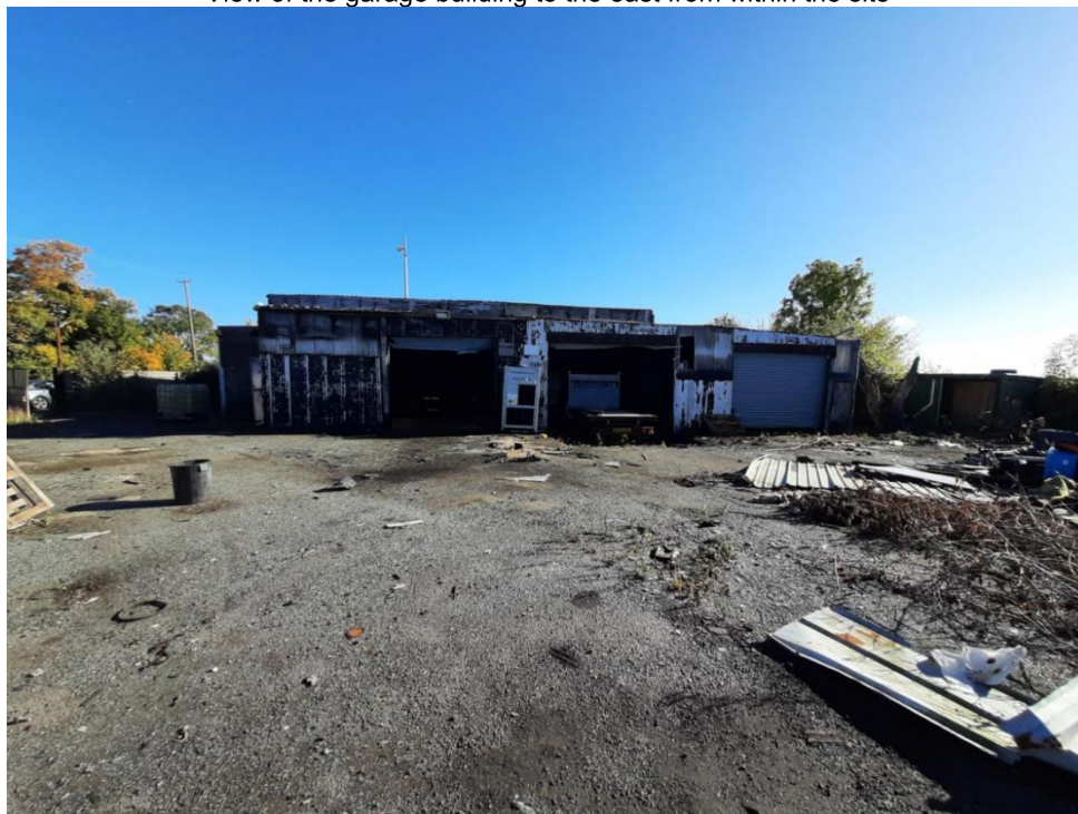
View of the garage building to the east from within the site
