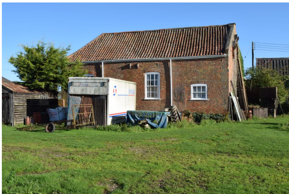
Looking north at the rear of the Grade II Listed Baptist Church.
