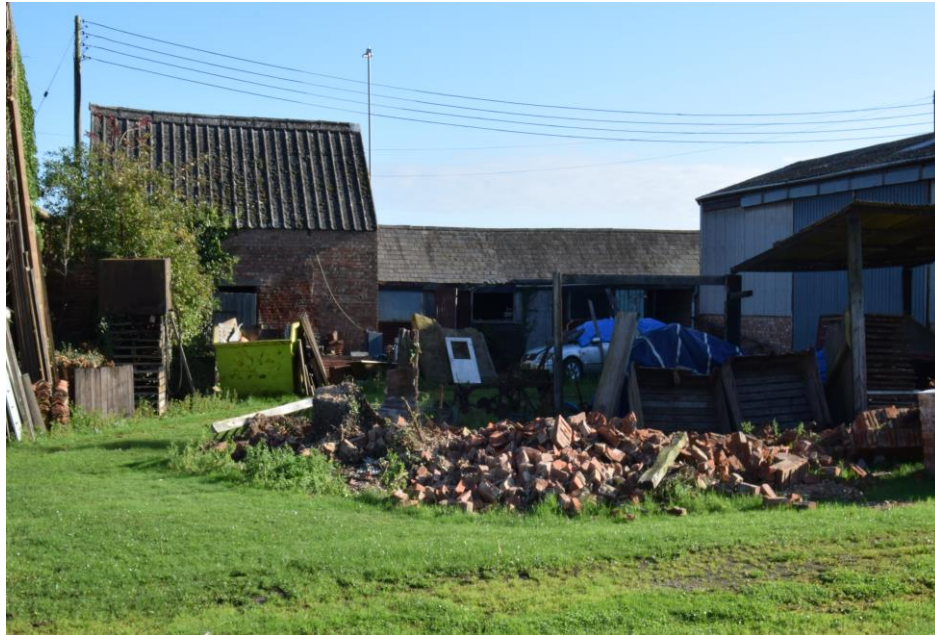
Looking at the range of agricultural buildings from the south.
