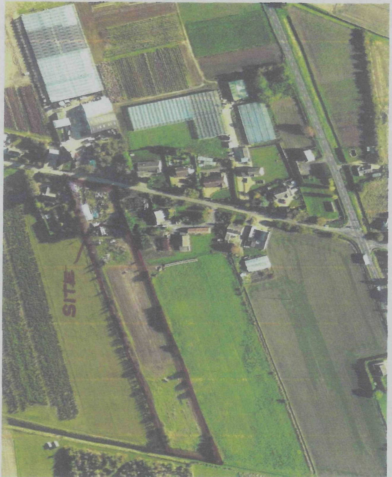
Picture of Site before Glasshouses erected.
