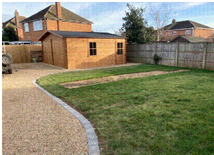
image of garage
