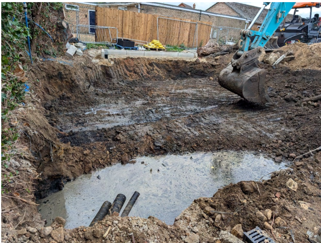
Photograph 10 – Former Pond Excavation
