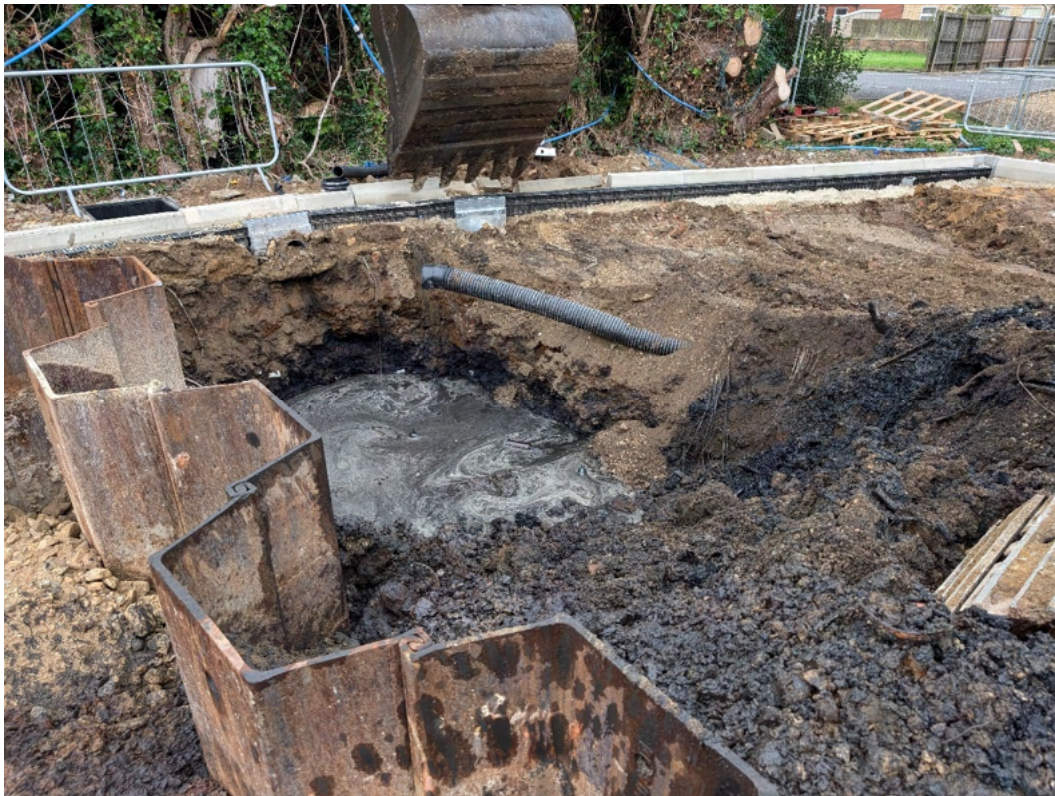
Photograph 9 – Former Pond Excavation
