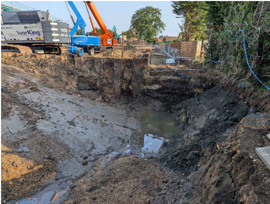
Photograph 11 – Former Pond Excavation
