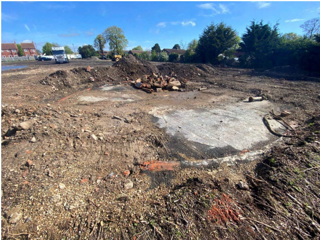
Photograph 7 – Former Sewage Works Concrete Pad
