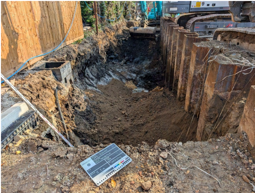
Photograph 13 – Former Pond Excavation
