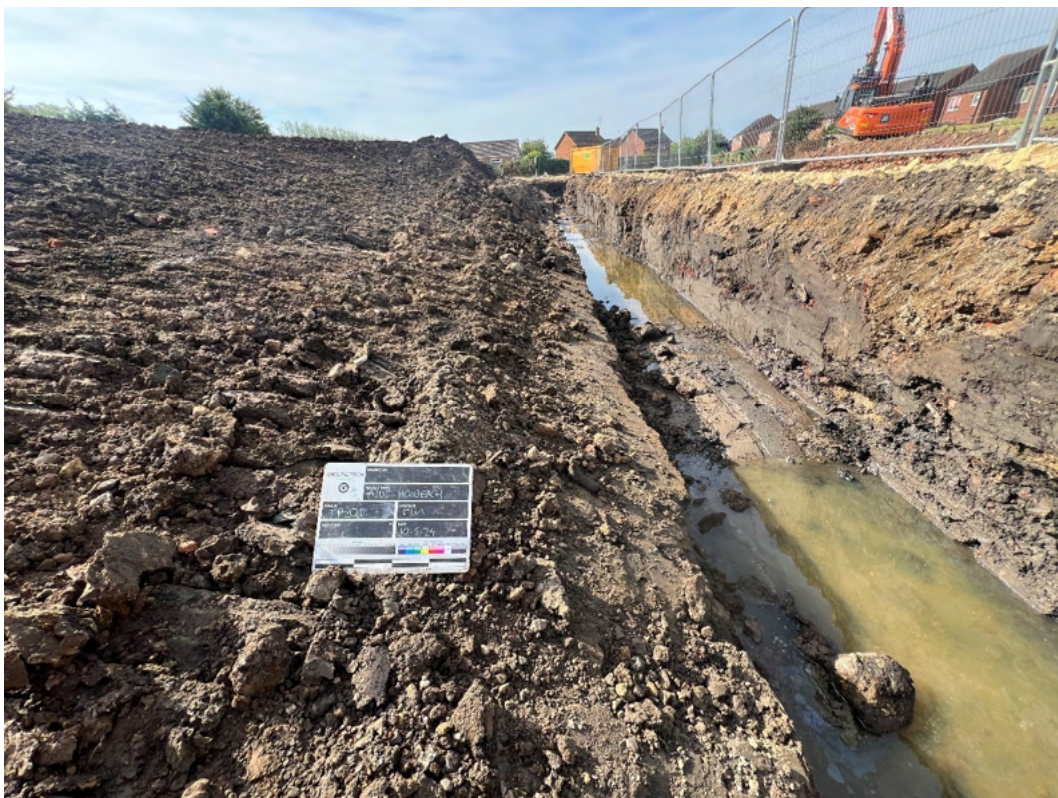
Photograph 8 – Former Drain Excavation
