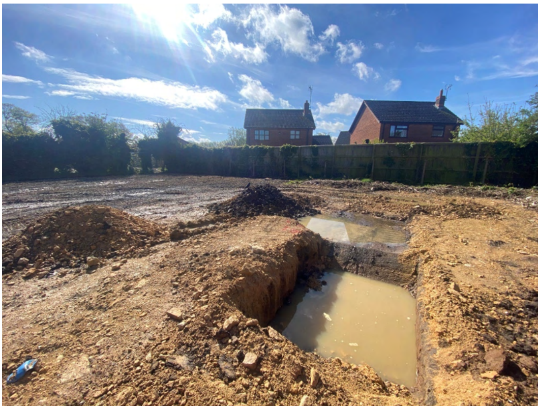
Photograph 6 – Groundwater Monitoring Excavation
