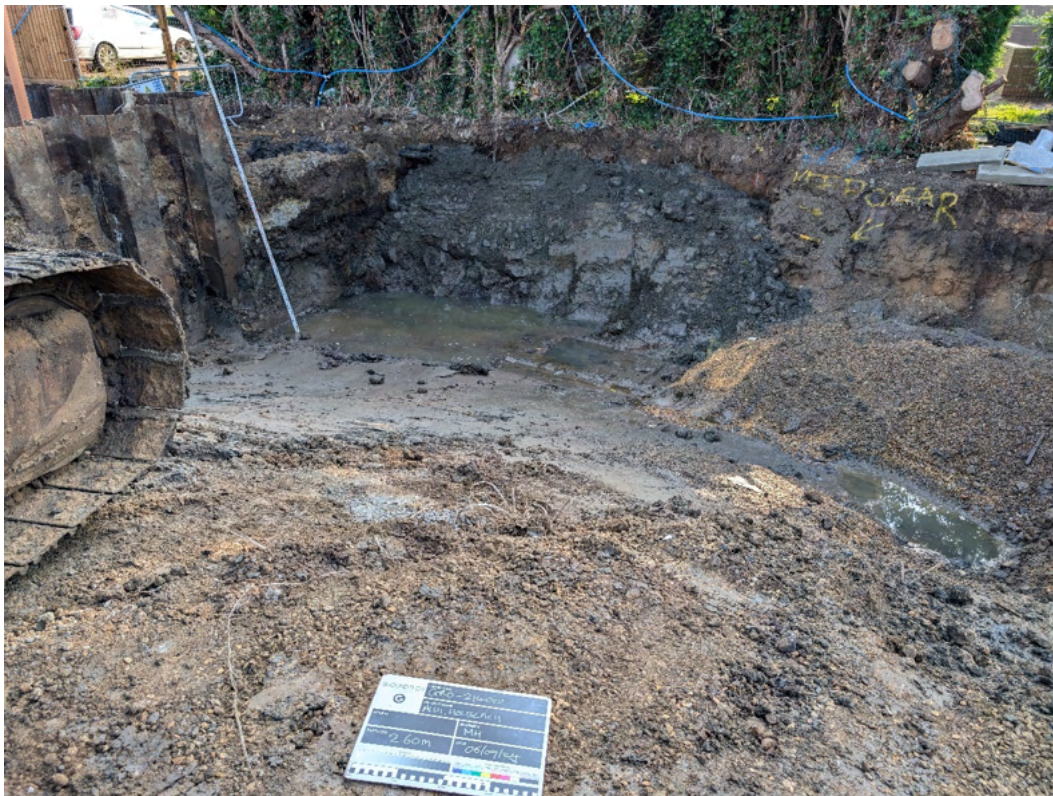
Photograph 12 – Former Pond Excavation
