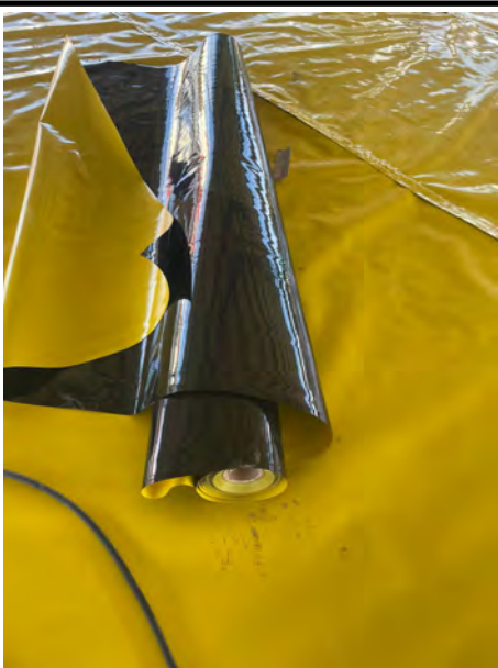
The JUTA GP5+ Gas Barrier being installed.
