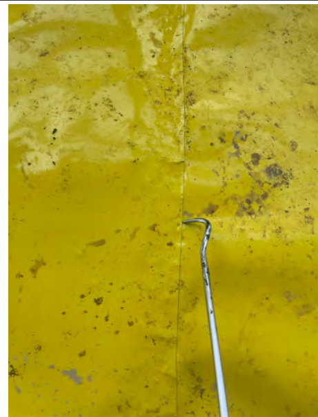
A pick and probe test being conducted upon a hand welded overlap.
