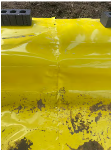
A hand welded overlap of the JUTA GP5+ Gas Barrier.
