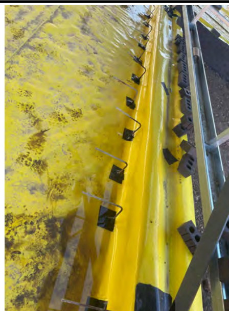
Steel Rebars sealed using Juta Titan Tank.
