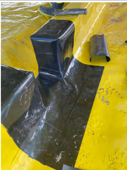
Details sealed with Juta Titan Tank.
