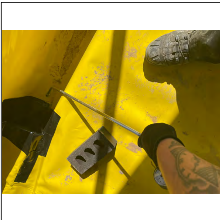
Air lance test on a corner.
