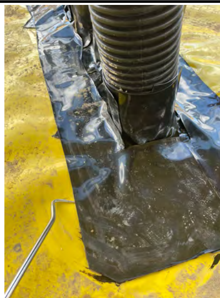
A pick and probe test being conducted upon a pipe penetration.
