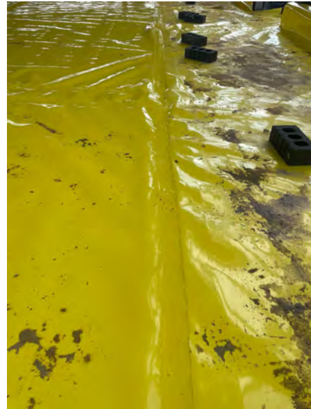
A dual welded overlap of the JUTA GP5+ Gas Barrier.
