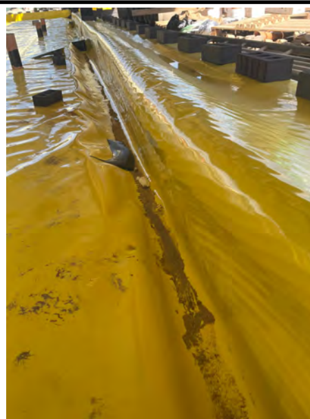
The JUTA GP5+ Gas Barrier installed tightly to the perimeter wall.
