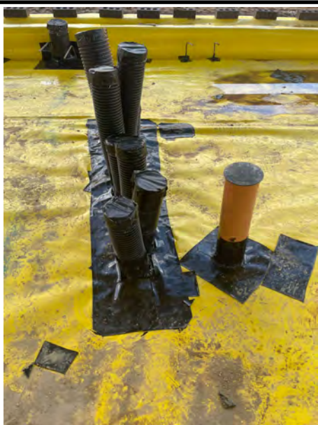
Sealed pipe penetrations.
