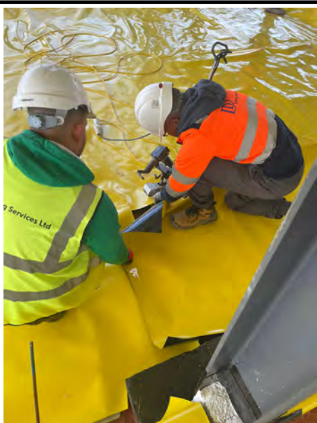
The installers welding overlaps of the JUTA GP5+ Gas Barrier.
