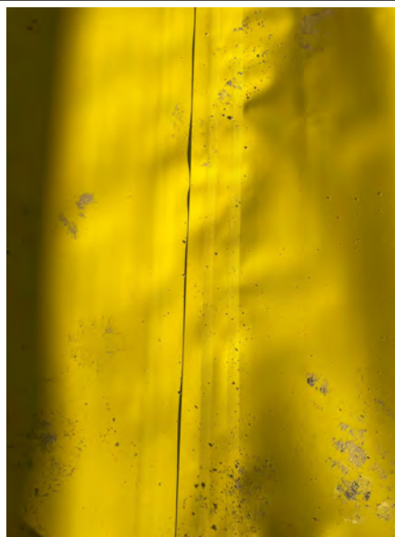
A dual welded overlap of the JUTA GP5+ Gas Barrier.
