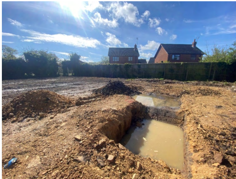
Trial Pit excavation to obtain groundwater sample (Wider Site)
