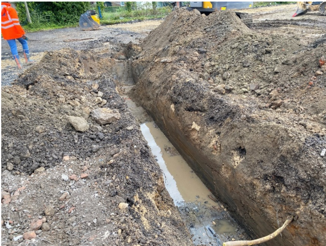
Trial Pit excavation to obtain groundwater sample (Former Pond Area)
