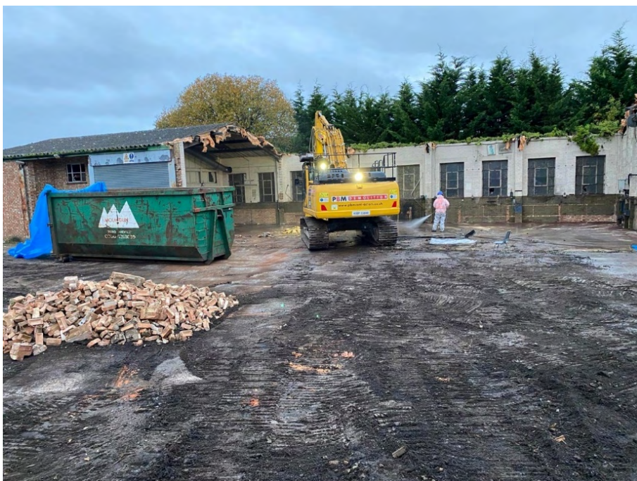
Demolition of Existing Structures (Former Depot)
