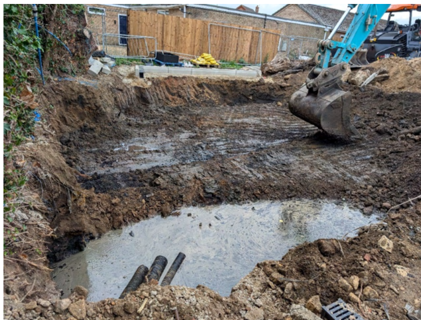
Delineation of former pond material (Initial Excavation)
