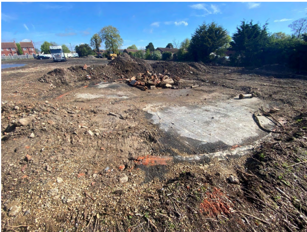
Former Sewage Works Concrete Pad
