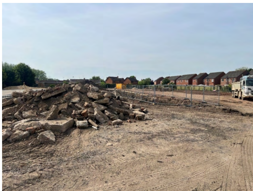
Former Drain Excavation (Relic chamber segments)
