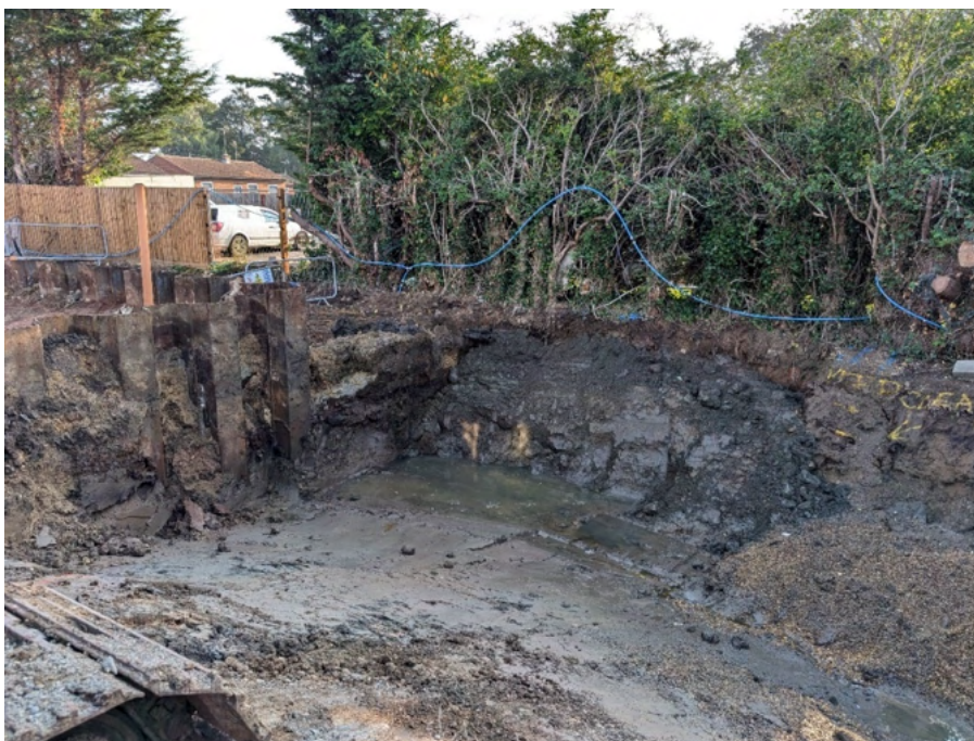
Delineation of former pond material (Final Excavation)
