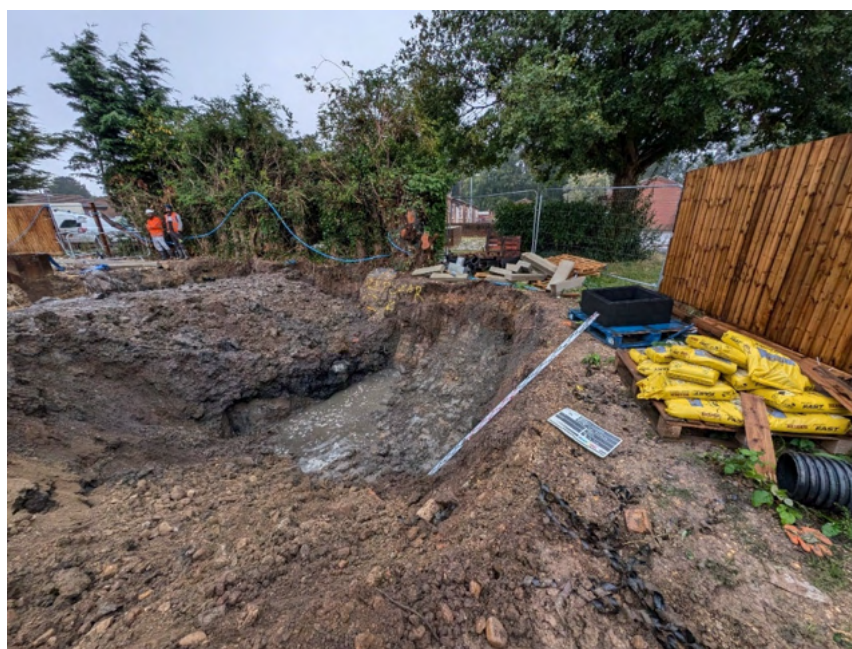
Delineation of former pond material (Staged Excavation)
