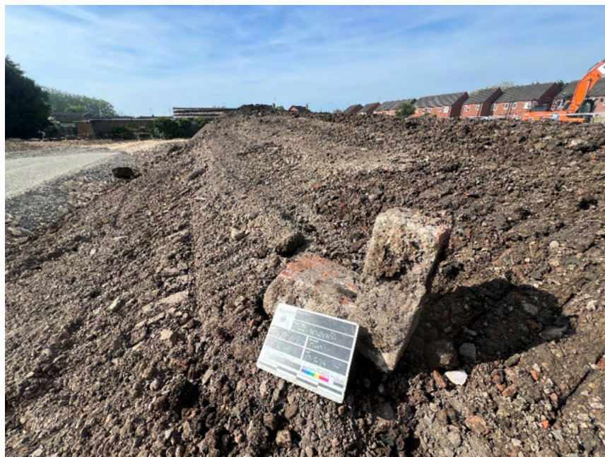
Former Drain Excavation (Relic chamber segments)
