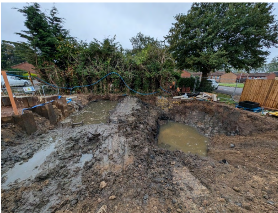
Delineation of former pond material (Staged Excavation)
