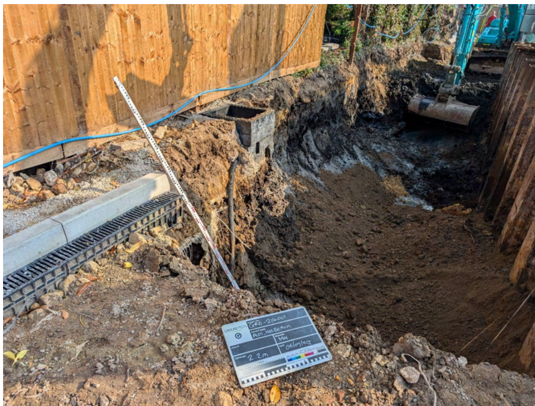
Delineation of former pond material (Final Excavation)
