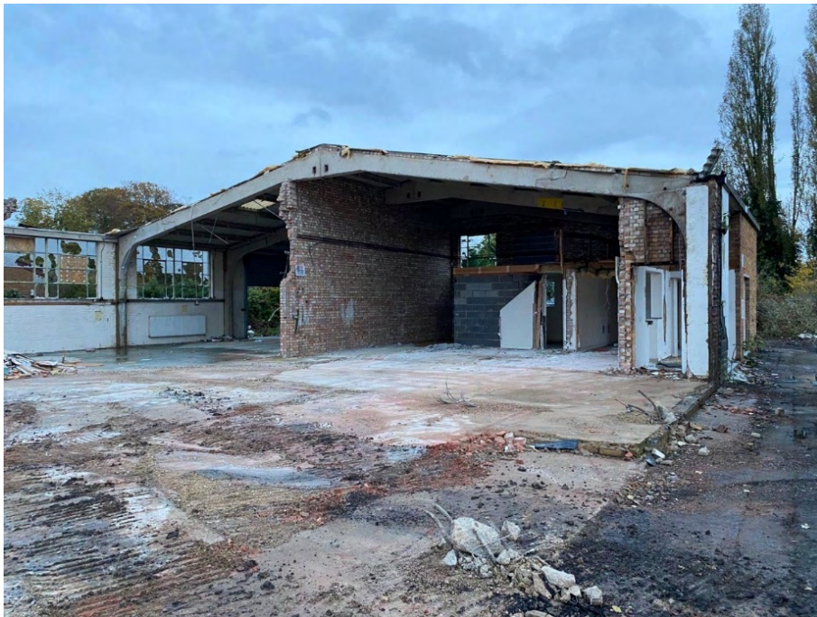
Demolition of Existing Structures (Former Gym)
