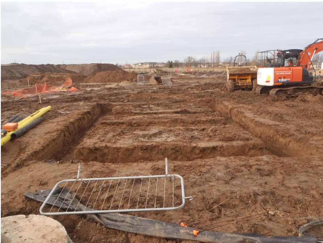
Plate 4. The completed Plot 15 footings, looking northwest
