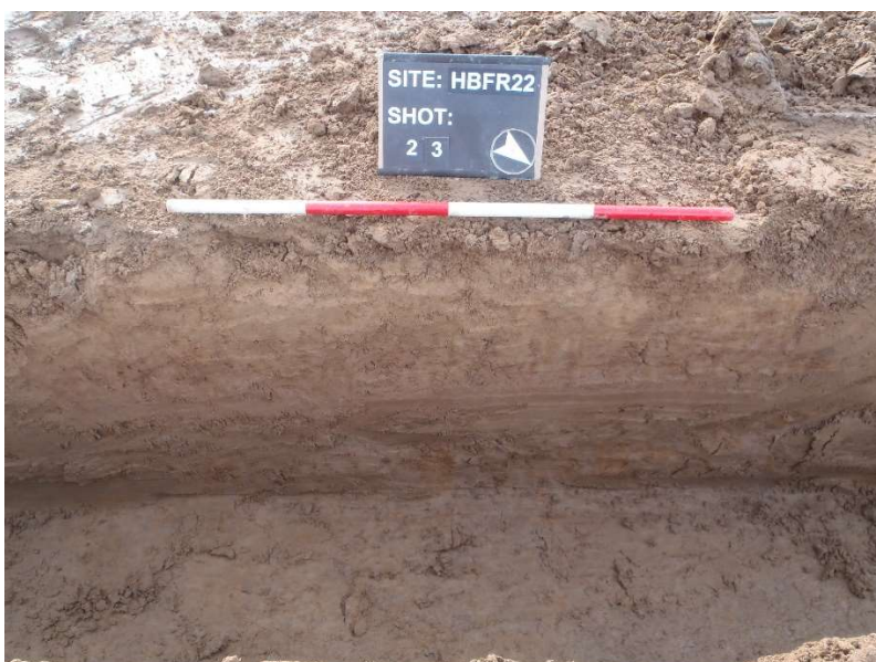
Plate 7. Plots 14/15 garage footings, representative Section 9, looking southwest
