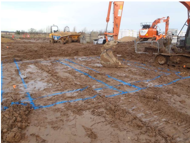
Plate 6. Pre-machining view of Plots 14/15 garage, looking north
