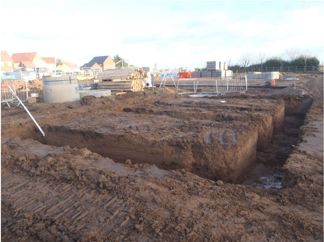
Plate 3. The completed Plot 14 footings, looking southeast
