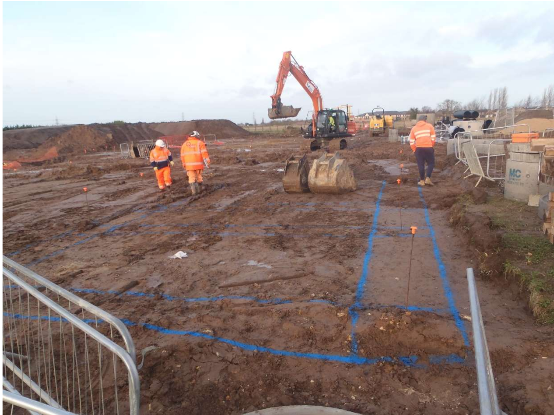
Plate 1. Pre-machining view of Plot 14, looking northwest
