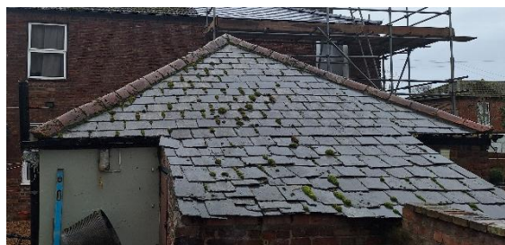
Rearmost roof – slate tiles
