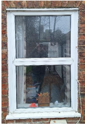
Existing aluminium framed windows
