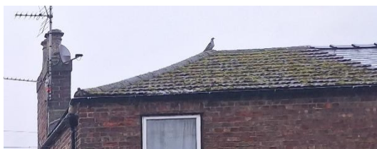
Main roof – concrete tiles
