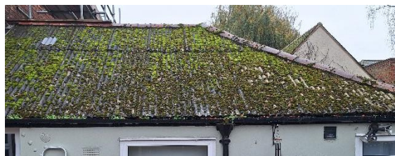
Rear roof – corrugated sheets
