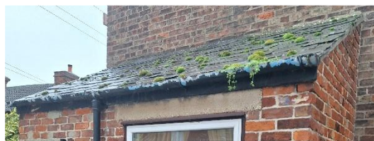
Side lean-to roof – slate tiles
