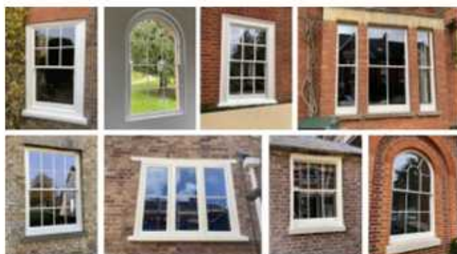
Left: Examples of heritage timber windows with retrofitted double-glazed units.
