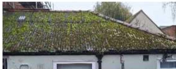
Rear roof – corrugated sheets
