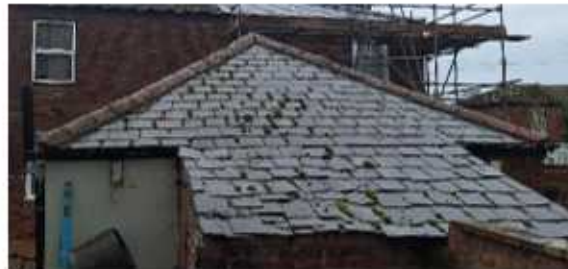
Rearmost roof – slate tiles
