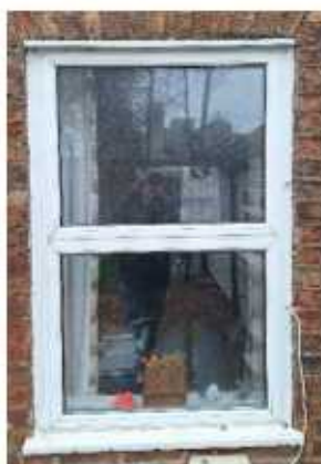
Existing aluminium framed windows
