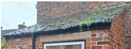
Side lean-to roof – slate tiles
