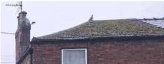
Main roof – concrete tiles
