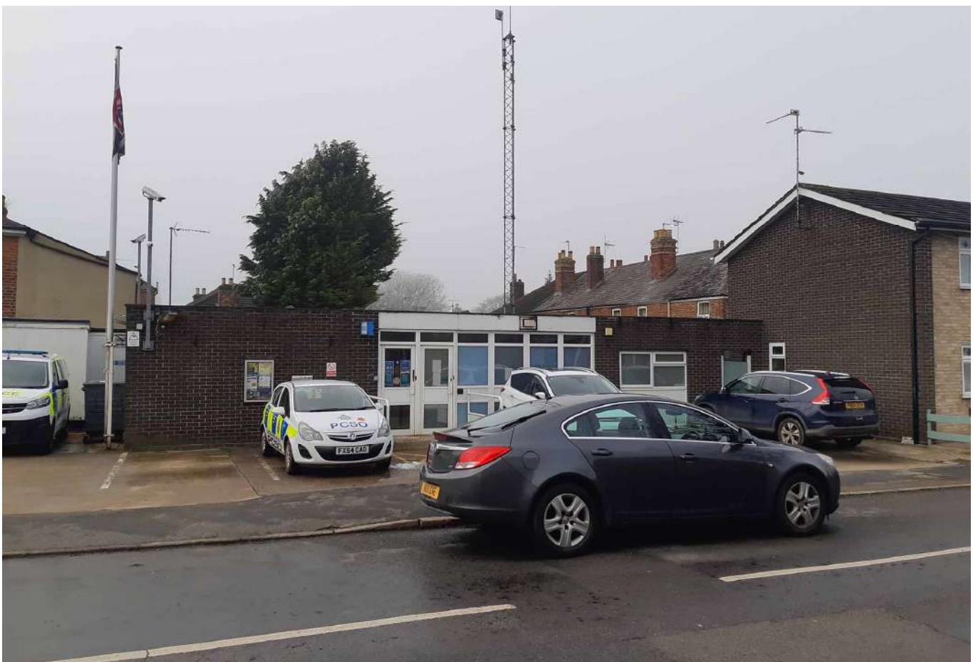
Figure 6: The east elevation of the existing police station and car parking viewed from Edinburgh Walk
