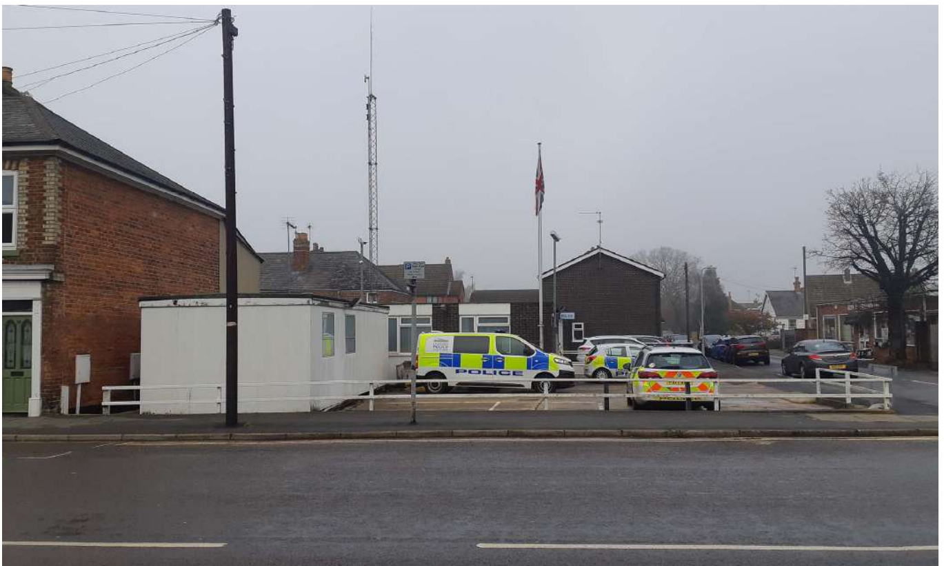
Figure 4: View north across the site from Fleet Street demonstrating the scale of the existing building in relation to the surrounding dwellings
