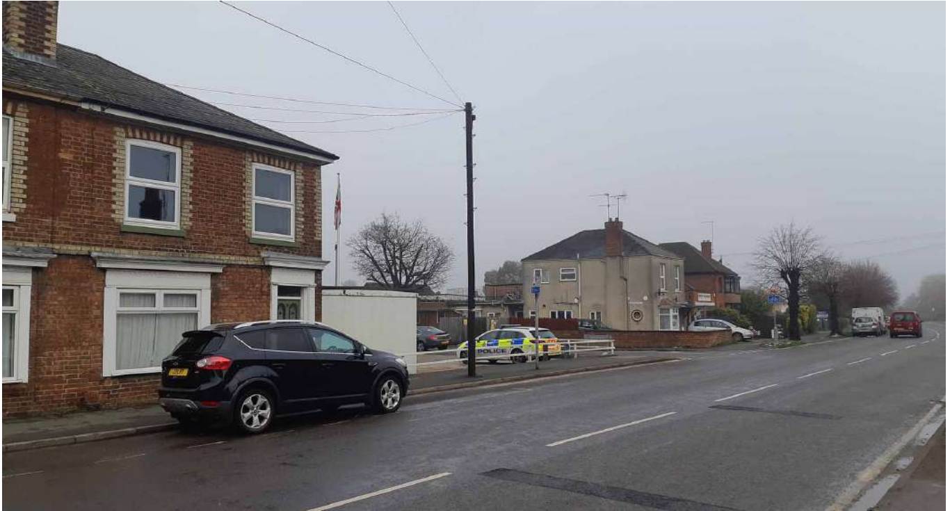
Figure 5: View north east along Fleet Street showing the street frontage and end elevation of the existing portacabin.
