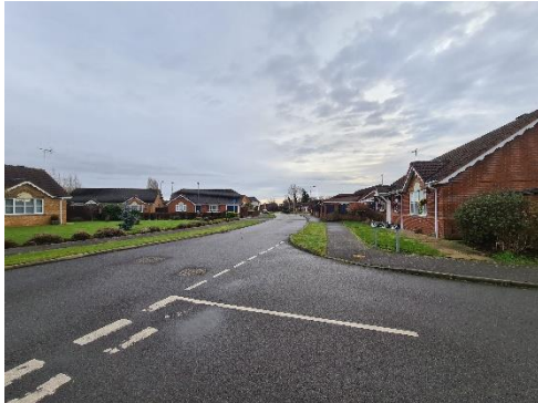
Photograph 1: Conditions on Kings Road
