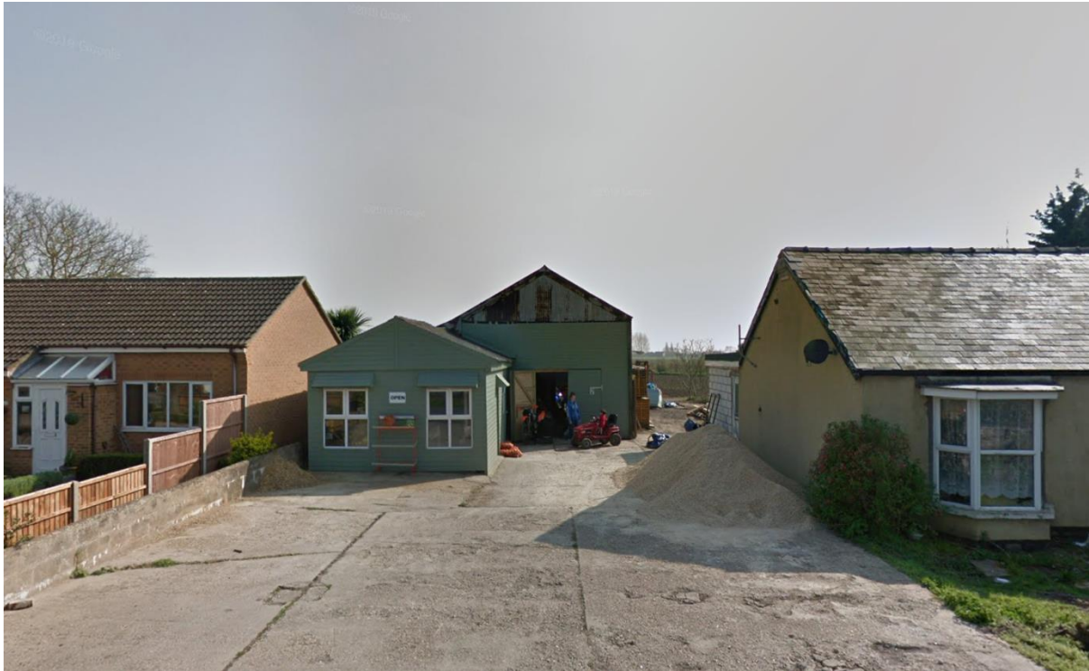
The site as viewed from the Main Road.
