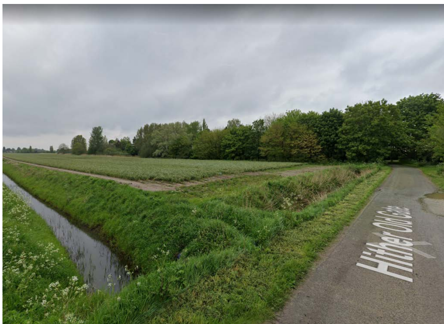
View of western boundary from Hither Old Gate
