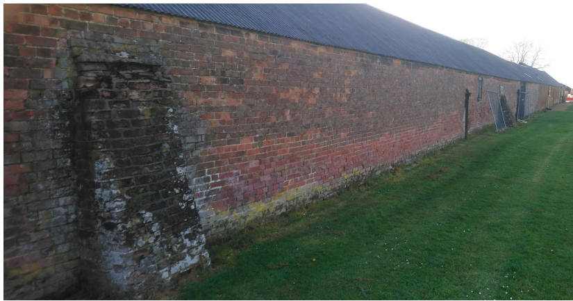
‘Barns 1’ at Leadenhall Farm, Holbeach St. Marks
